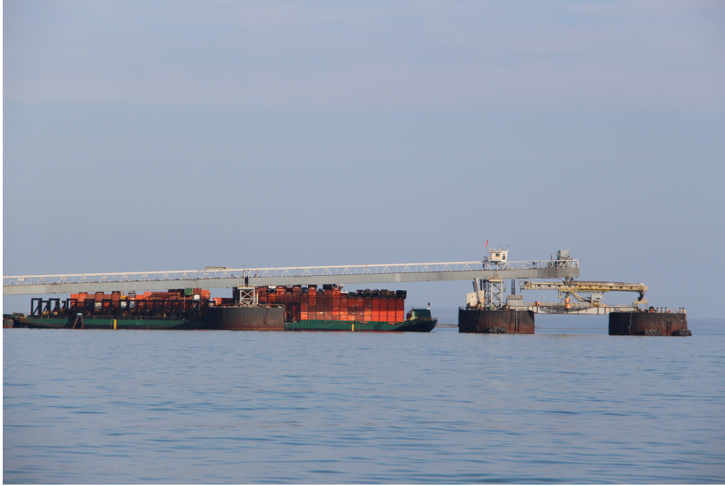
Figure 2.1. DeLong Mountain Shipping Terminal (aka “Red Dog Port Site”)
