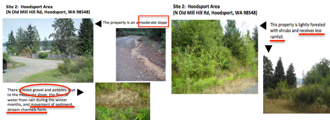
Figure 4-7 Site Photographs and Information
