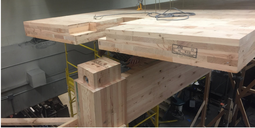
Figure 2.3: All-Wood connection test between CLT Elements for the Framework Building(Lever Architects, Portland University, Portland, OR, USA; 2017)
