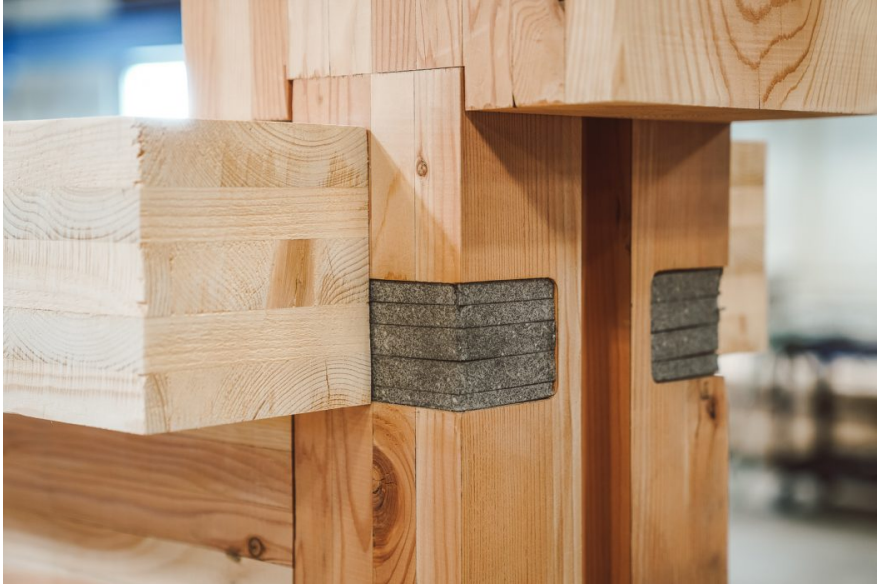
Figure 2.2: All Timber Connection with intumescent strips for the Heartwood Building (Atelier Jones, TimberLab, Seattle, WA, USA; 2022)
