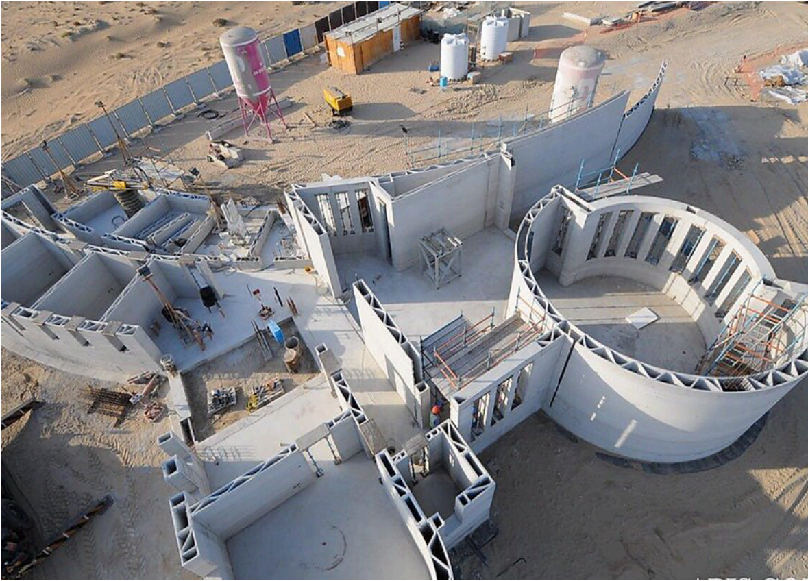
Figure 4.14: Dubai Municipality Administrative Building by Apis Cor (apis-cor.com).
