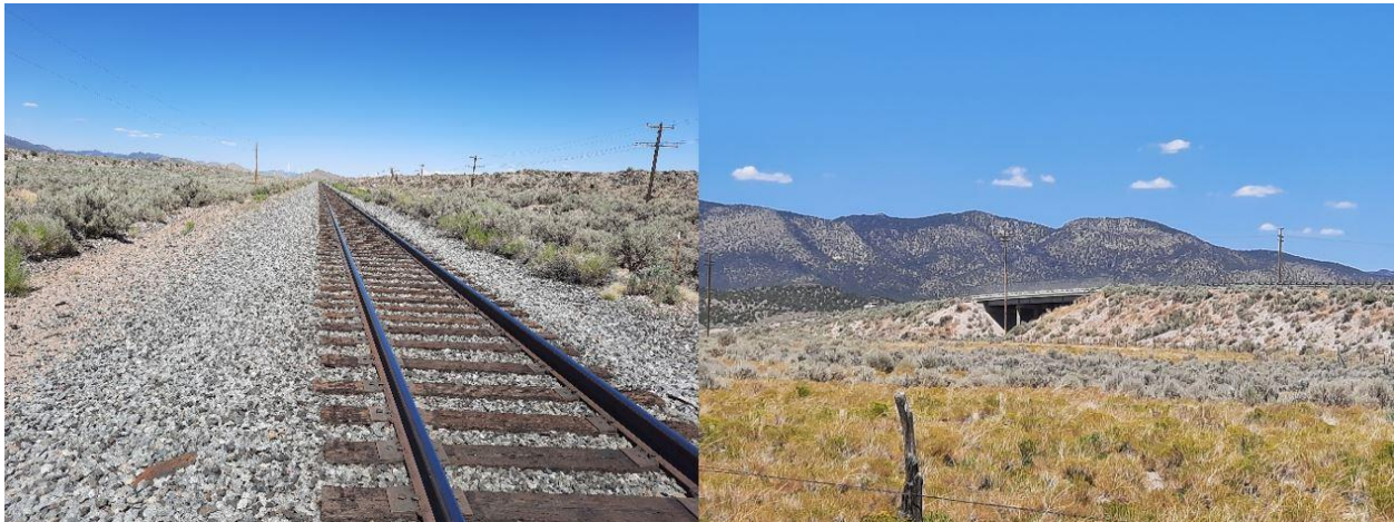
Figure 3-49: Anthropogenic dams at the Panaca Summit/Modena bottleneck; raised railroad bed and highway overpass.
