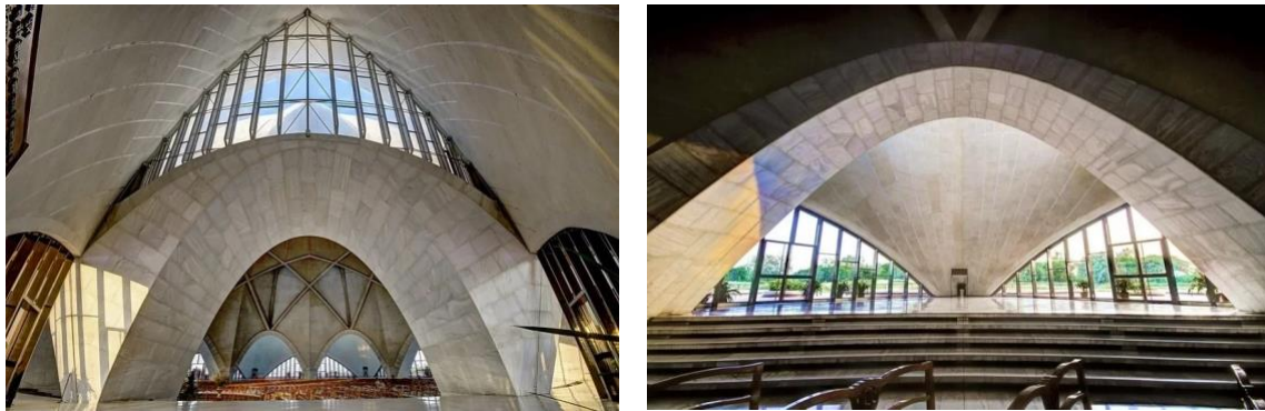
Image 3.9 Inner fold between petals installed with glass for light (Source: Bahá'í House of Worship)
