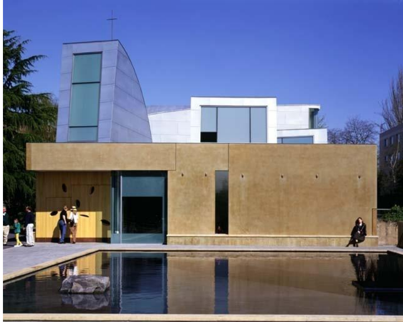
Image 1.2 Chapel of St Ignatius, Seattle, USA (Source: ArchDaily)
