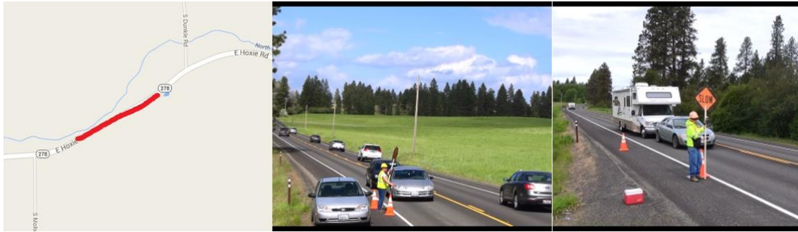
FIGURE A-2 Location and site photos for work zone #2
