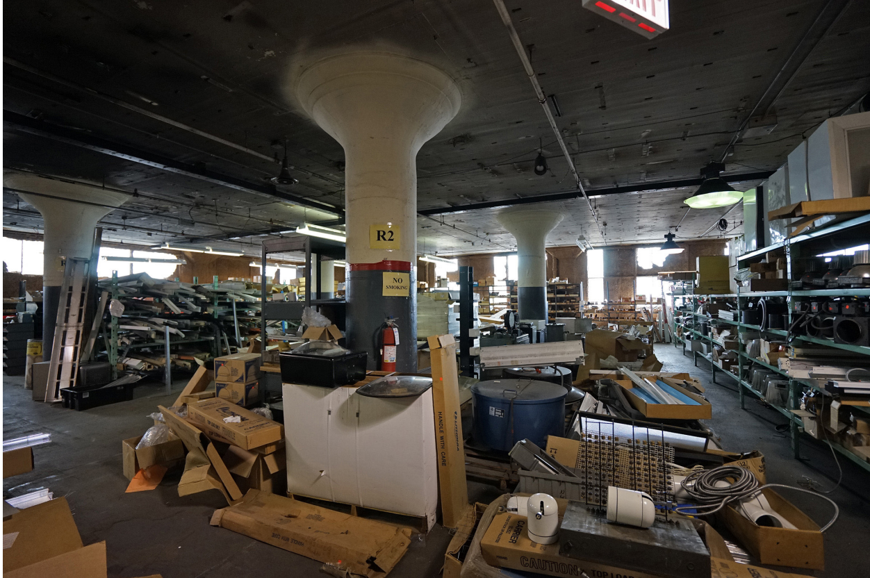
Fig. 4.6 Windows on the third floor of Delco Plant 2 showing the effect of spray insulation. Photo: April 2015, by author.
