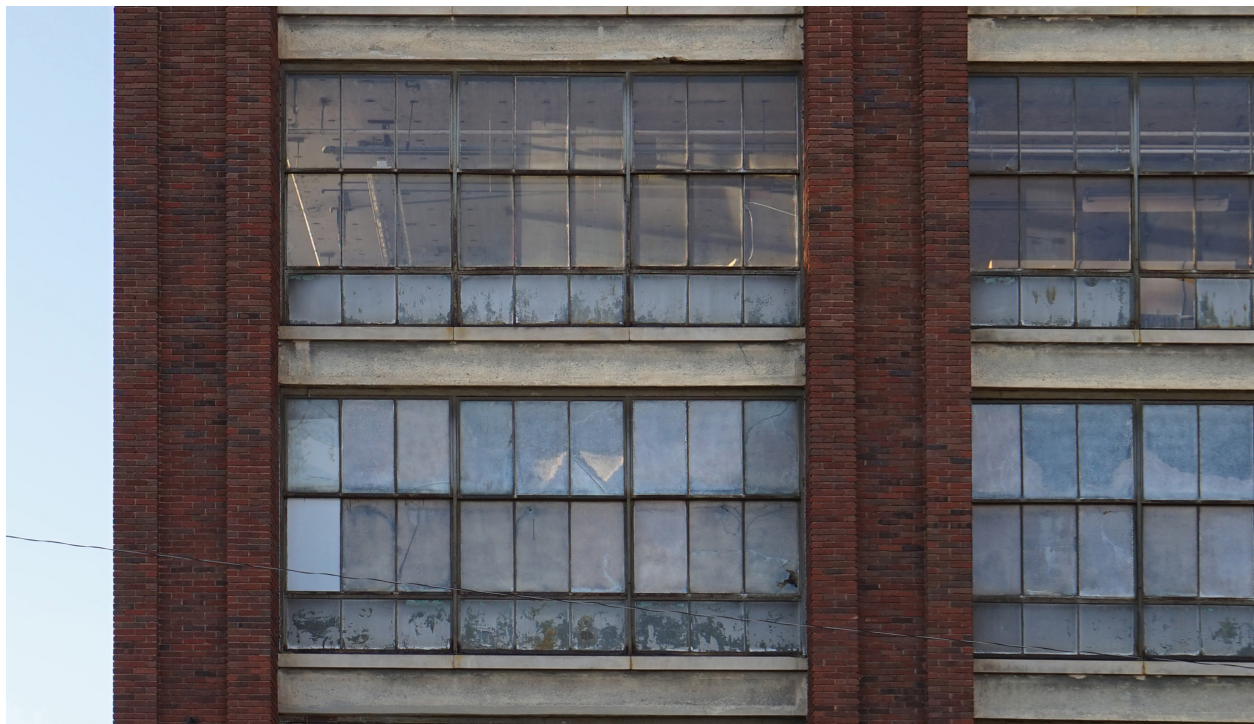
Fig. 3.61 Window detail of the third and fourth floors on the south side of the southwest corner of the 1915 portion of Delco Plant 2. Photo: April 2015. by author
