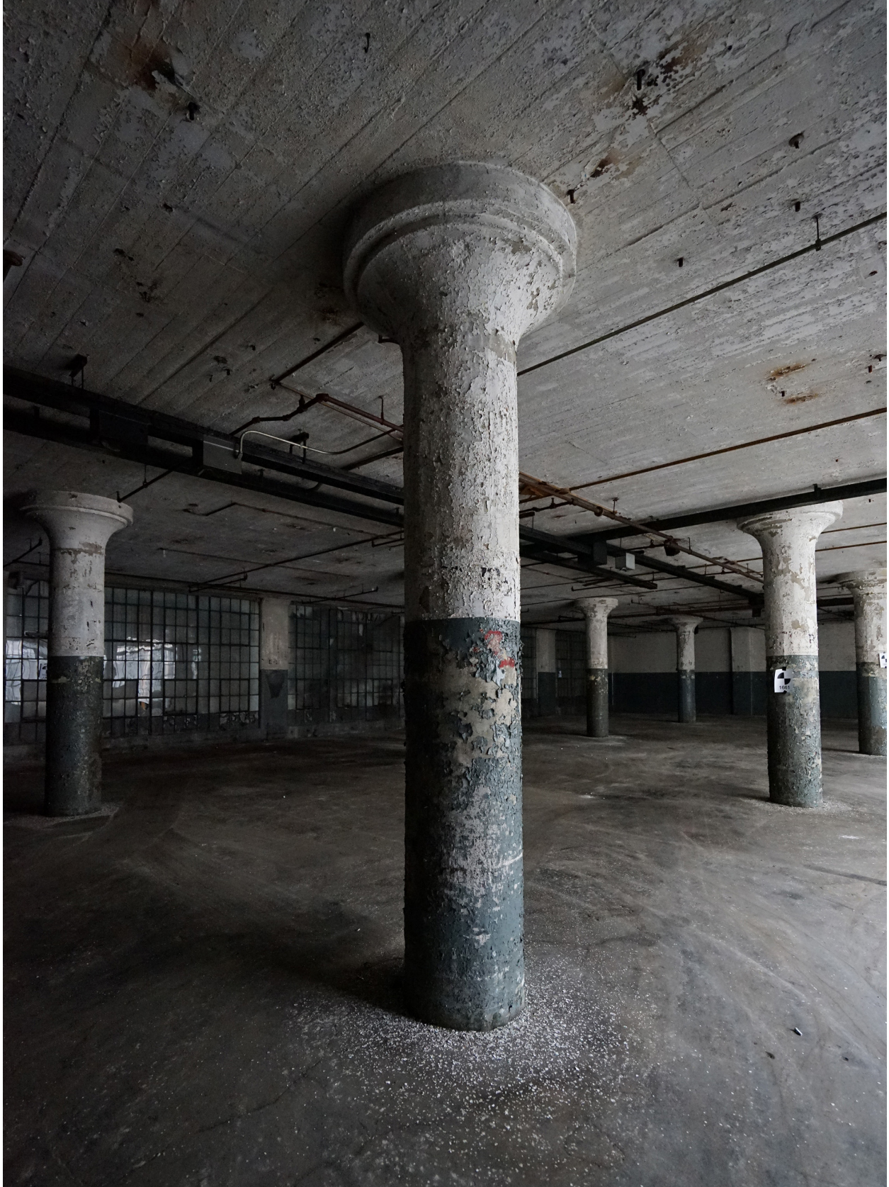
Fig. 3.44 Typical interior mushroom column from the third floor demonstrating the flat slab two-way structural system. Photo: April 2015, by author.
