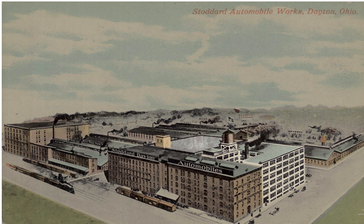
Fig. 3.10 The two new concrete frame buildings of the Dayton Motor Car Company, highlighted in a c. 1908 postcard. The 1907 building with the light well is to the right, and the 1908 building that remains today is to the left. Image from the Dayton Postcard Collection at the Dayton Metro Library. (Shading added.)
