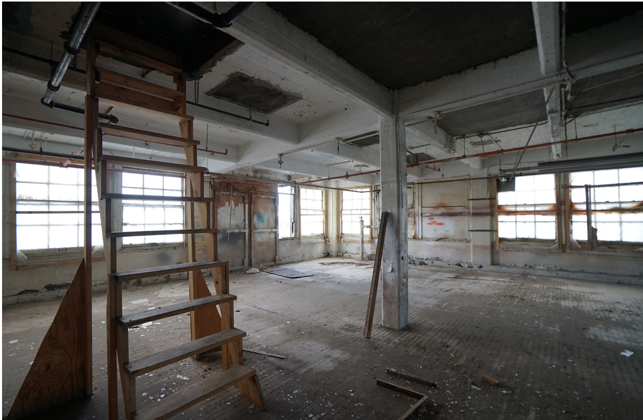
Fig. 3.19 Sixth floor detail showing ceiling patches, wood floor, and typical column width. Photo: April 2015, by author.
