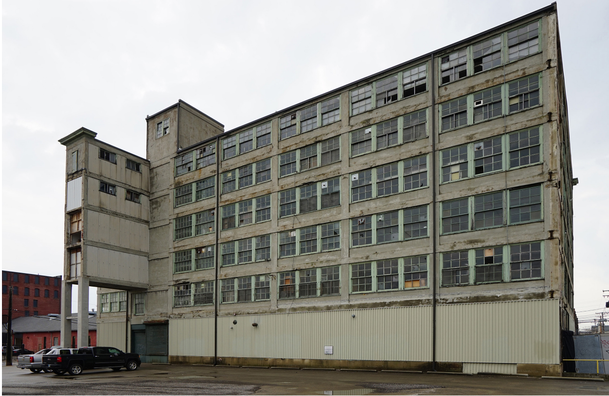
Fig. 3.20 North facade showing former passage to masonry buildings, infill at the elevator location, and an irregular window pattern. Photo: April 2015, by author.
