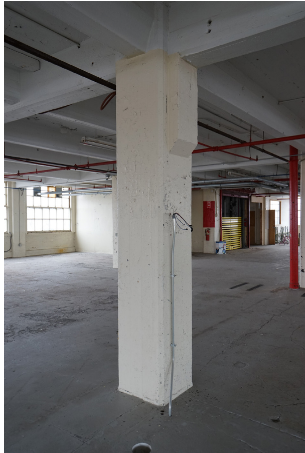
Fig. 3.23 Typical square column and connection to floor girders on third floor. Photo: April 2015, by author.
