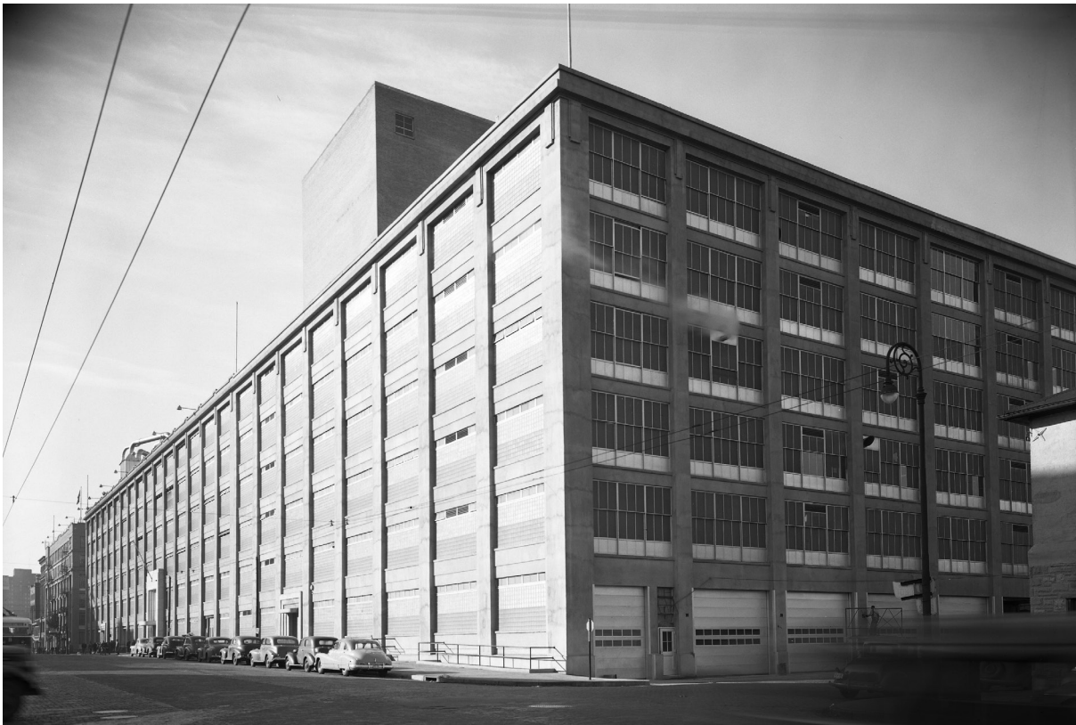
Fig. 3.35 Delco Plant 3 was built in 1923 and demolished in 1981. Photo: 1948, from the collections at Dayton History.
