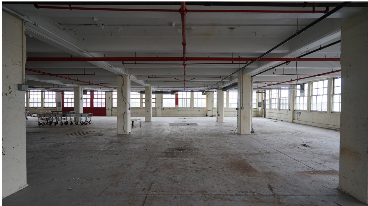
Fig. 3.24 Typical bay from third floor showing girder system and building systems. Photo: April 2015, by author.
