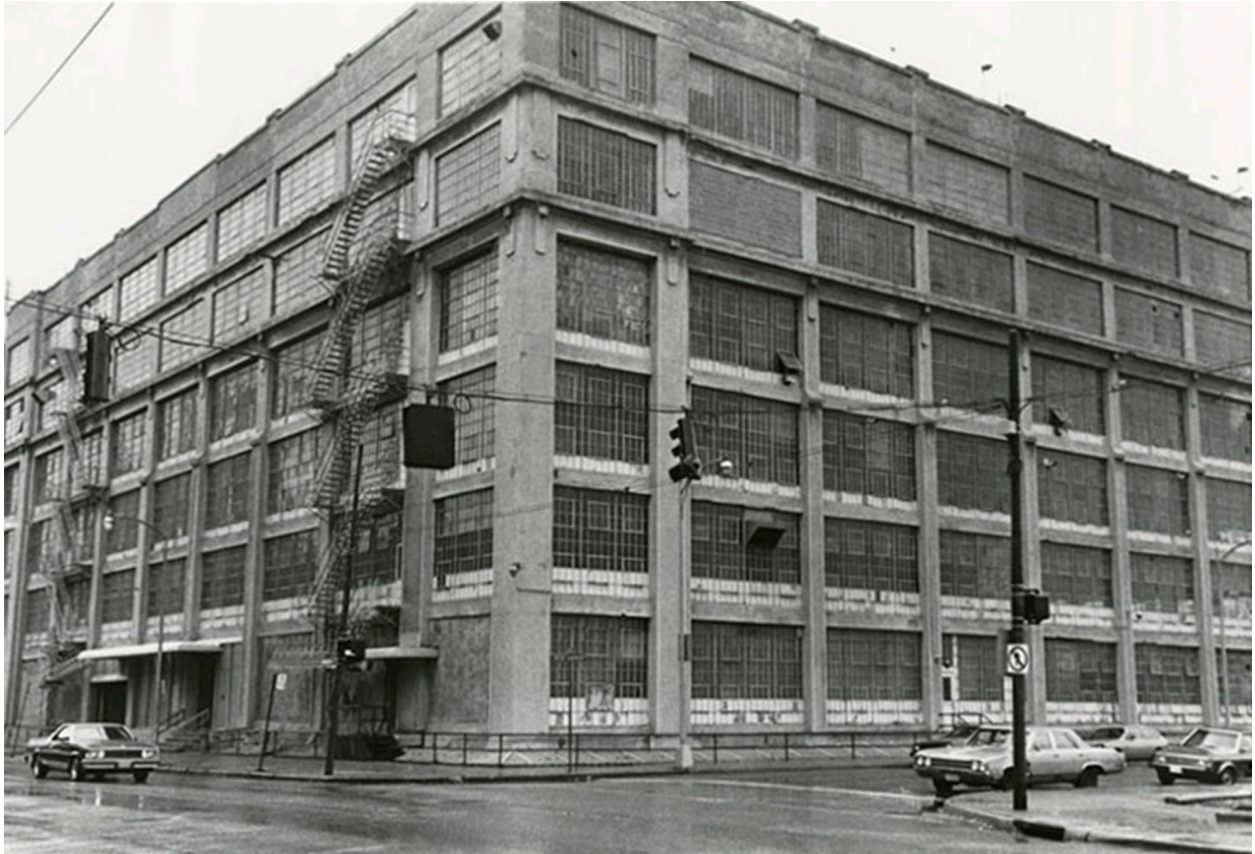
Fig. 3.39 Delco Plant 1. Photo: c. 1970 from Wright State University.
