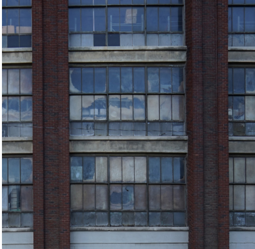
Fig. 3.63 Spray insulation can be seen covering windows on the second and third floors from the exterior. Photo: April 2015, by author.
