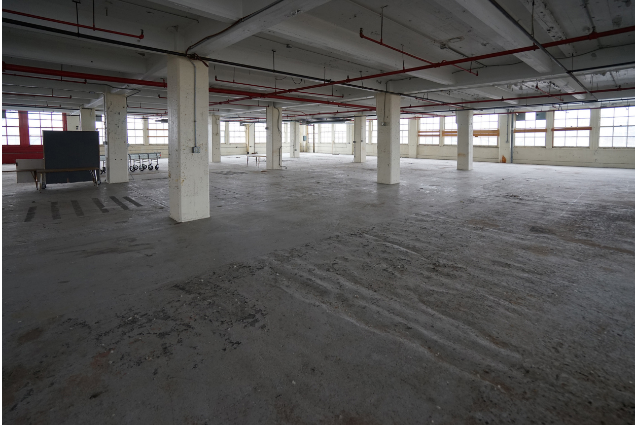
Fig. 4.2 Third floor of the Dayton Motor Car Company building showing its open floor plan. Photo: April 2015, by author.
