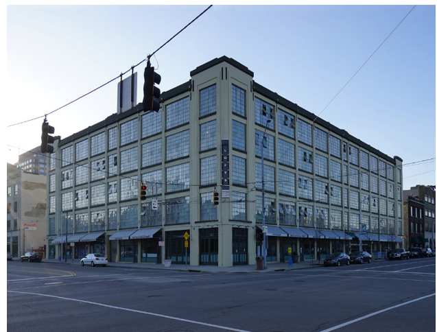
Fig. 3.4 Schenck & Williams, Beaver Power Building #1, southeast corner, Dayton, OH, 1910. Photo: April 2015, by author.
