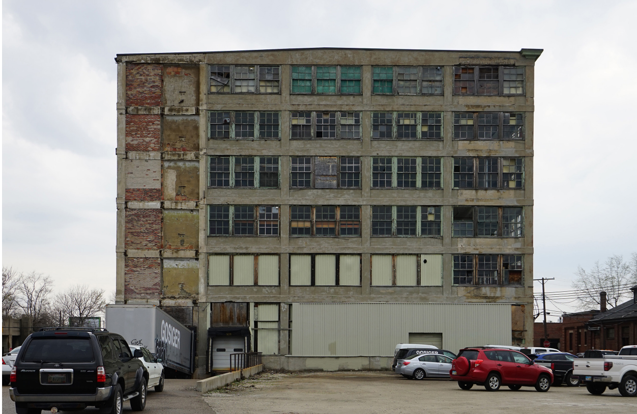
Fig. 3.21 West facade showing infill. Photo: April 2015, by author.
