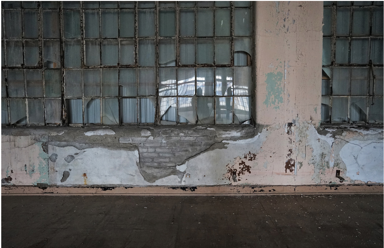
Fig. 3.46 Interior of perimeter wall on sixth floor showing concealed masonry construction. Photo: April 2015, by author.
