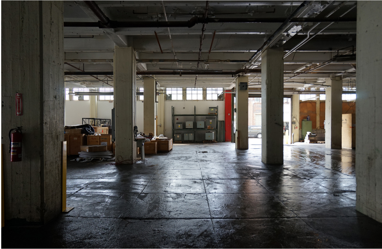
Fig. 3.18 Typical bay on the ground floor showing column thickness. Photo: April 2015, by author.
