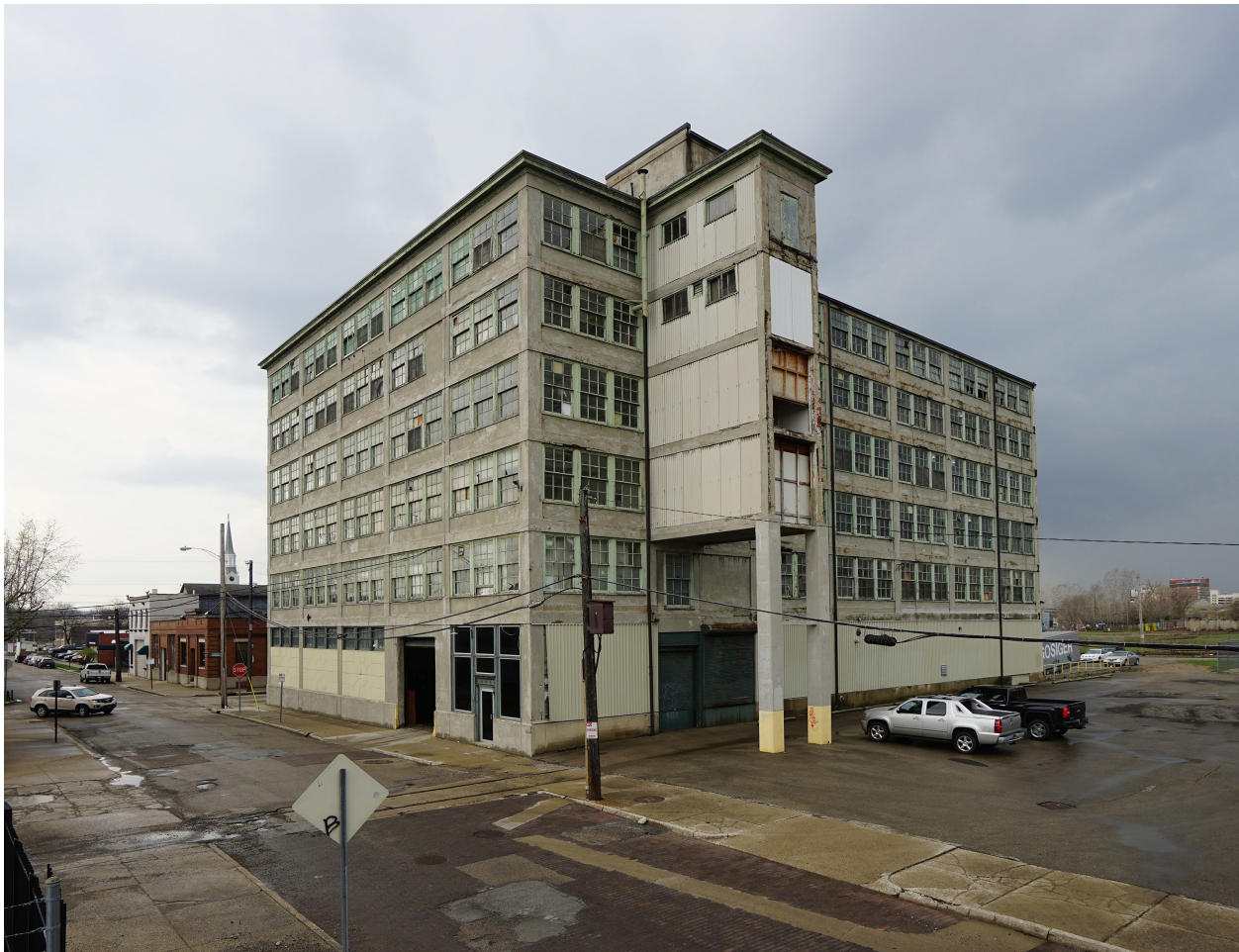
Fig. 3.9 [Keppele Hall Company?] Dayton Motor Car Company, northeast corner, 1908. Photo: April 2015, by author.
