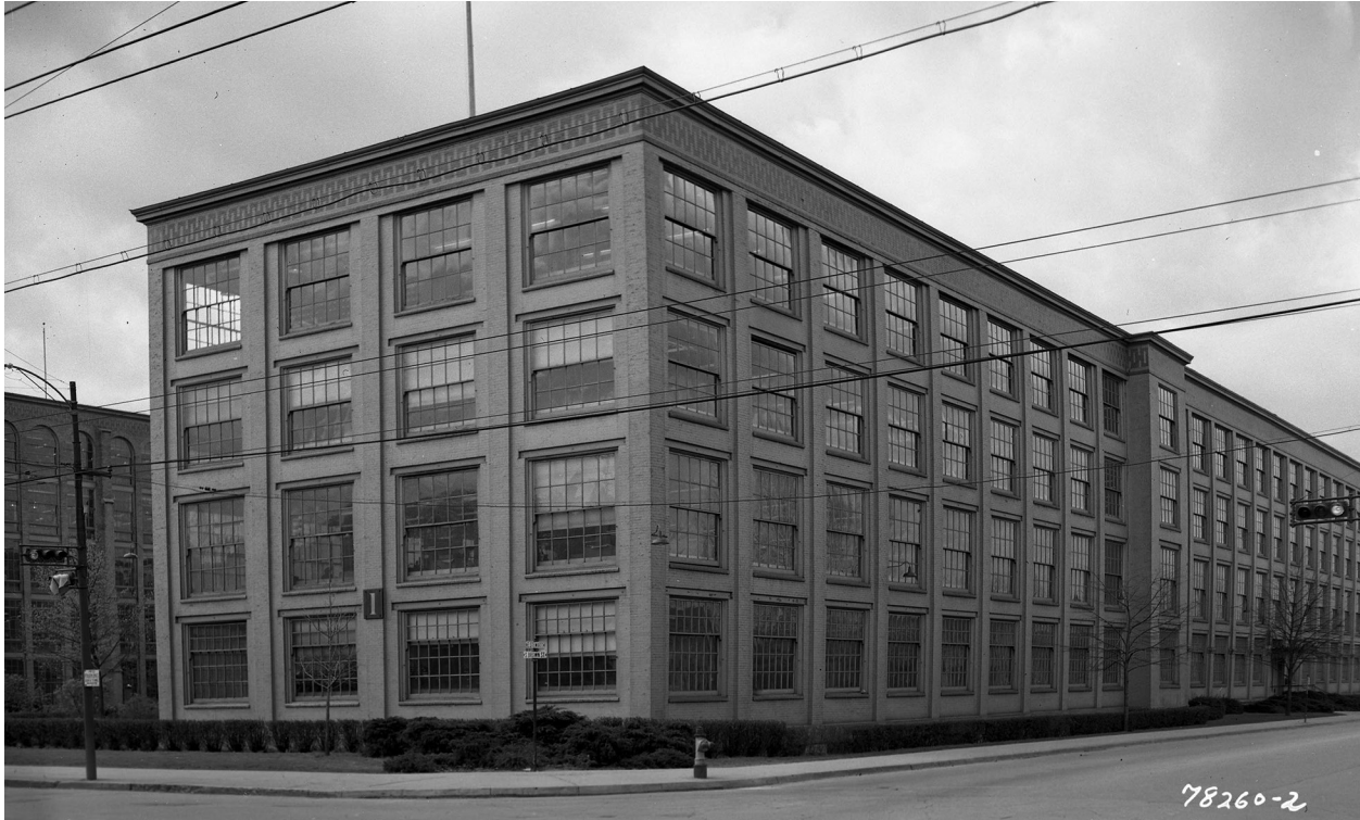
Fig. 2.9 Building #1 of the National Cash Register Company, designed by architect Frank Mills Andrews c. 1887. The factories were known for their large windows that provided ample lighting and ventilation for the comfort and safety of their workers. Photo: 1953, from the collections of Dayton History.
