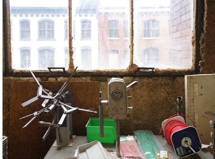
Fig. 3.64 Detail of spray insulation on a third floor window in the northeast part of the 1915 building, April 2015. Original window elements appear to be in good condition. Photo by author.
