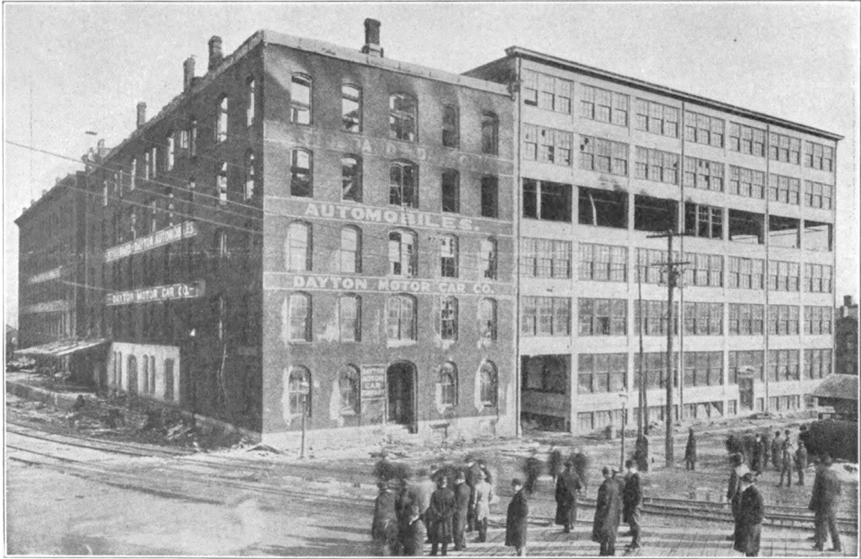
Fig. 3.15 Fire damage at the Dayton Motor Car Company in February, 1908. Photo from Insurance Engineering , 1908, v. 15, p. 373.
