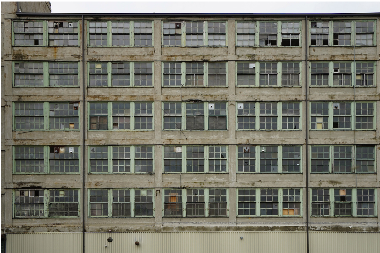
Fig. 3.25 North elevation of the building at 15 McDonough Street showing window condition and details as well as overall facade concrete-to-glass ratio. Photo: April 2015, by author.
