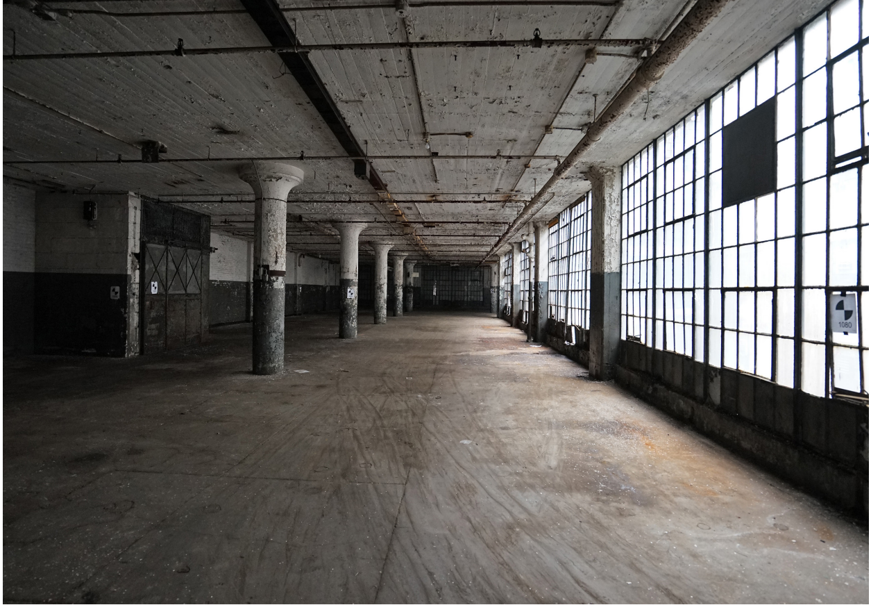
Fig. 4.5 Third floor of Delco Plant 1 showing concrete frame and expansive space. Photo: April 2015, by author.
