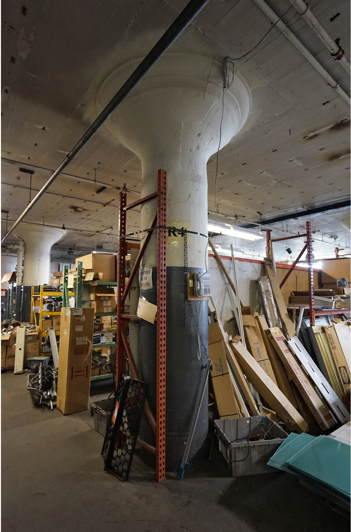
Fig. 3.59 Typical interior column on third floor. Photo: April 2015, by author.
