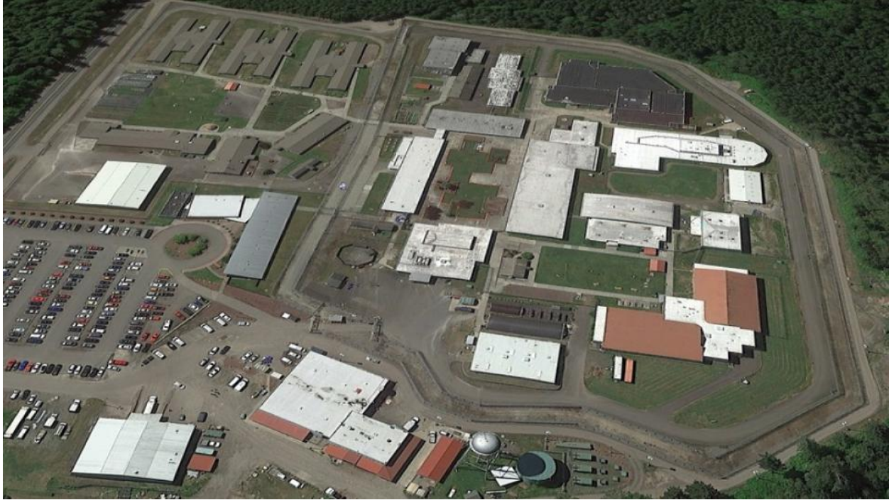
Figure 1. Washington Corrections Center for Women from above. Source: Washington Department of Corrections
