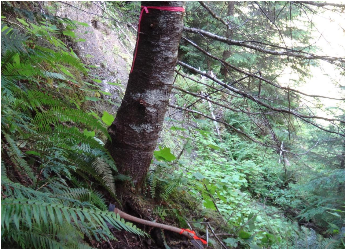
Figure 5. A conifer growing next to a shallow landslide on the toe of the deep-seated landslide.
