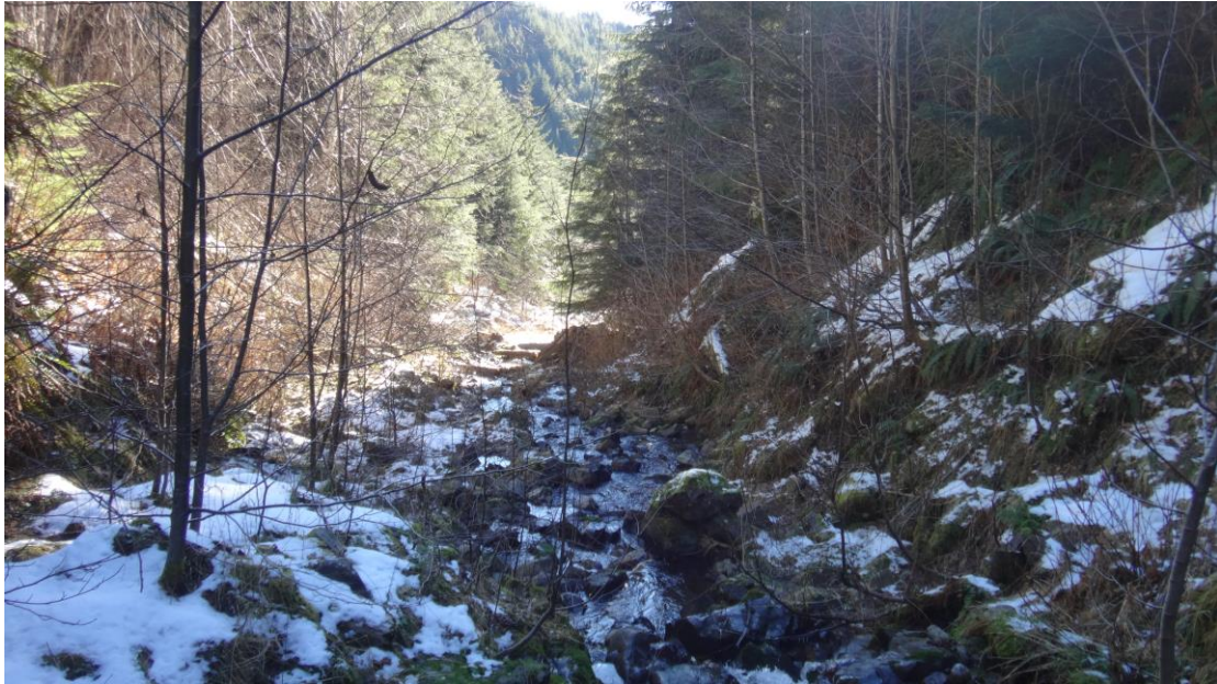
Figure 3. Looking downstream at the channel adjacent to landslide toe. Right channel wall has been scoured up to 3 meters above the channel bed. Young alders are growing on the channel bed and channel walls.
