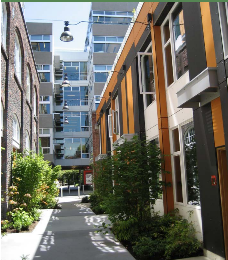
Changes in materials and textures combined with sizeable recesses and alterations in building height create visual massing breaks.
