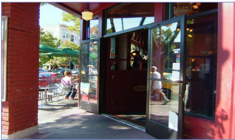
A well-marked, articulated building entrance that is oriented to the sidewalk and provides overhead cover.
