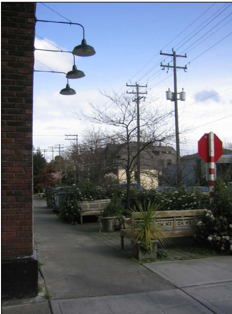
An example of drop lighting attached to a building.
