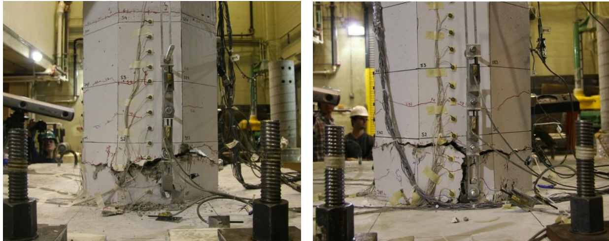
Figure 2.13 Dominant crack planes formed in columns made with fiber reinforced concrete shells (from Finnsson 2013).
