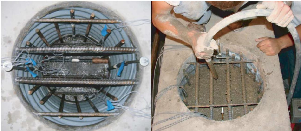
Figure 2.3: Pocket connection (from Restrepo et al. 2011)
