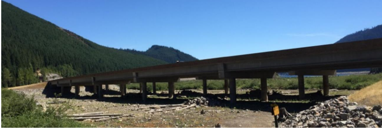
Figure C.2 Gold Creek Bridge (from Stephens 2016)
