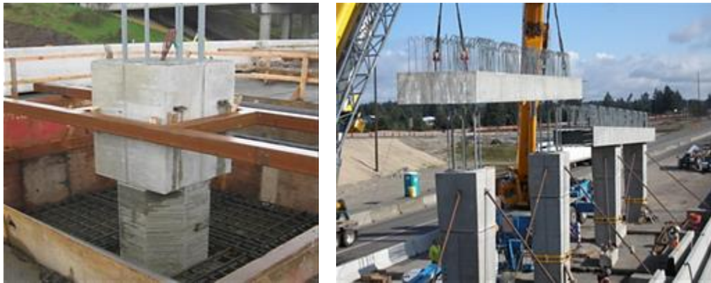
Figure 3.1 Construction of a non-prestressed, precast bridge bent (from Khaleghi et al. 2012).
