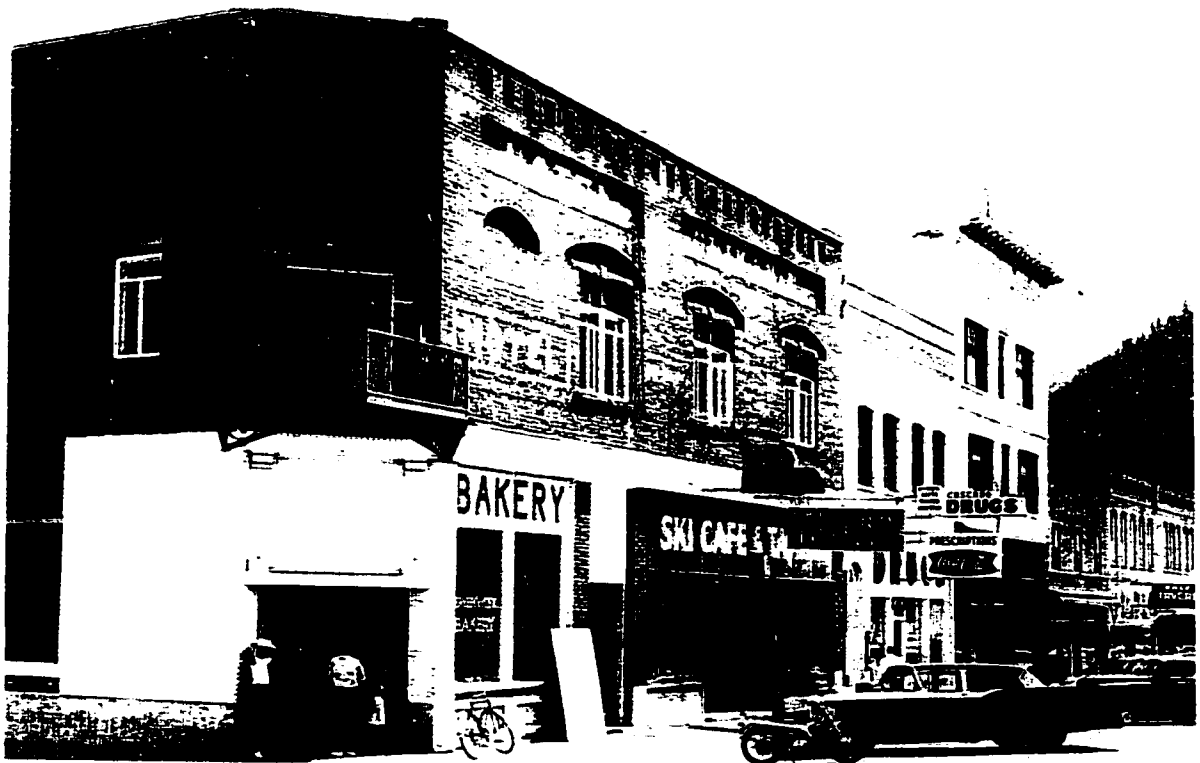
Figure 2.6: Edelweiss Hotel at start of renovation in 1966. From Price 68.
