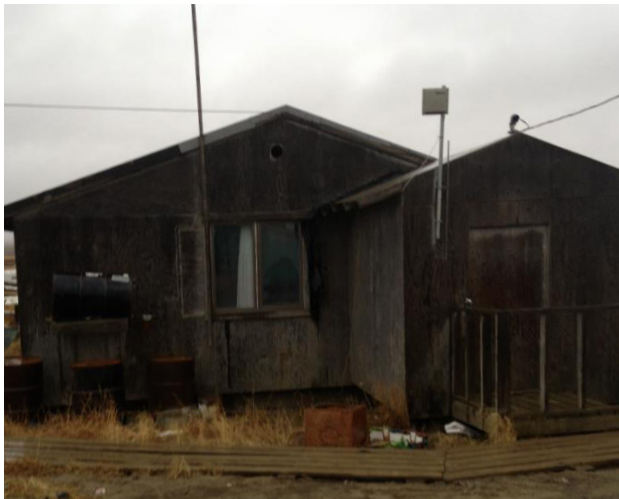
FIG 4. The front of a home in Toksook Bay, Alaska.
