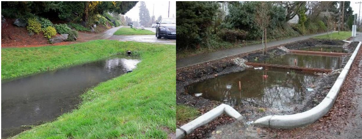
Graphic 16. Poorly designed and maintained rain gardens can become mosquito habitat
