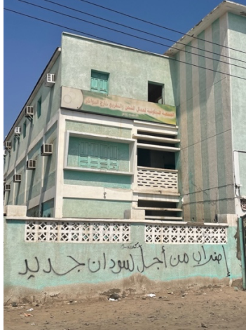
Figure 14: The Shipboard Cargo Loading and Unloading Workers Association Building in Portsudan
