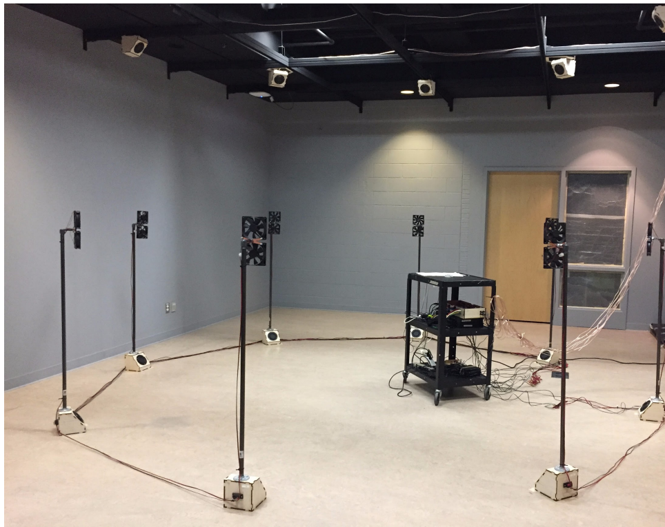
Figure 5.30. Installation and Testing
