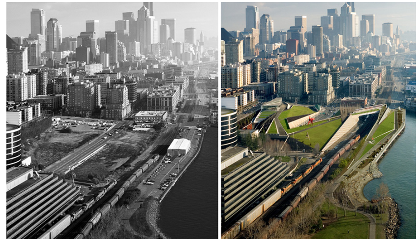
Figure 40: OSP before and after
