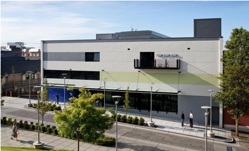
Figure 36: RFM renovated exterior
