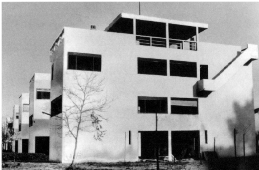
Figure 11: Housing at Pessac as originally built, 1924
