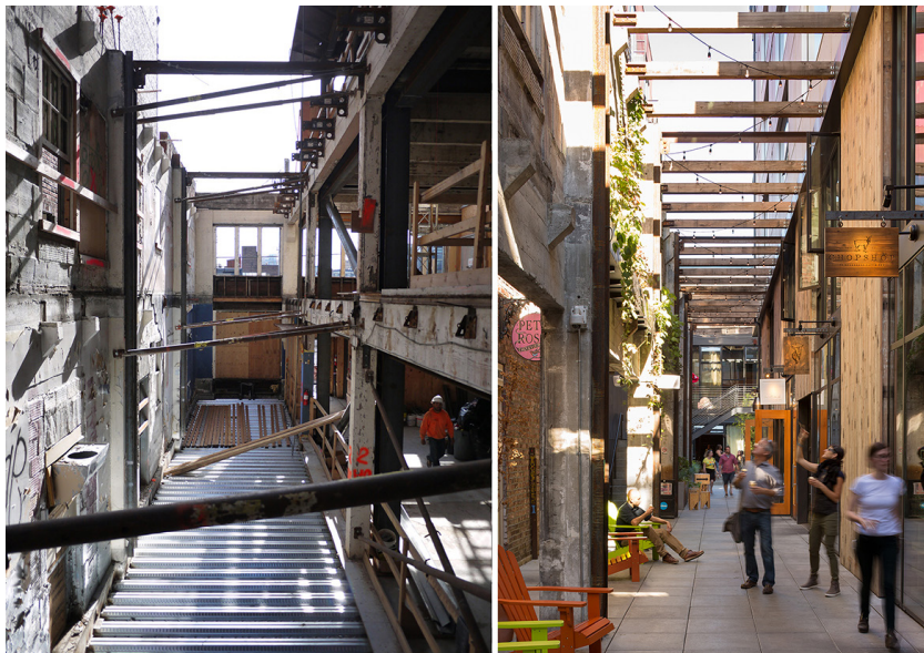
Figure 23: Chophouse Row Alley, during and after construction, 2015
