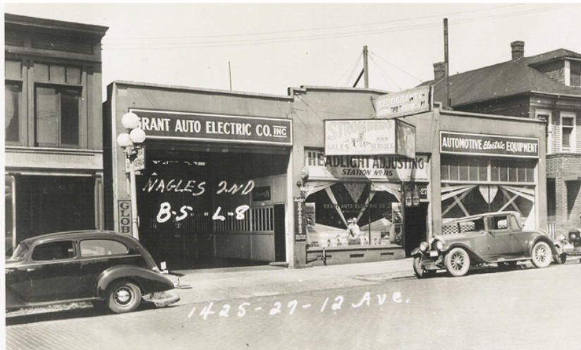
Figure 20: The Piston and Ring Building, before renovation
