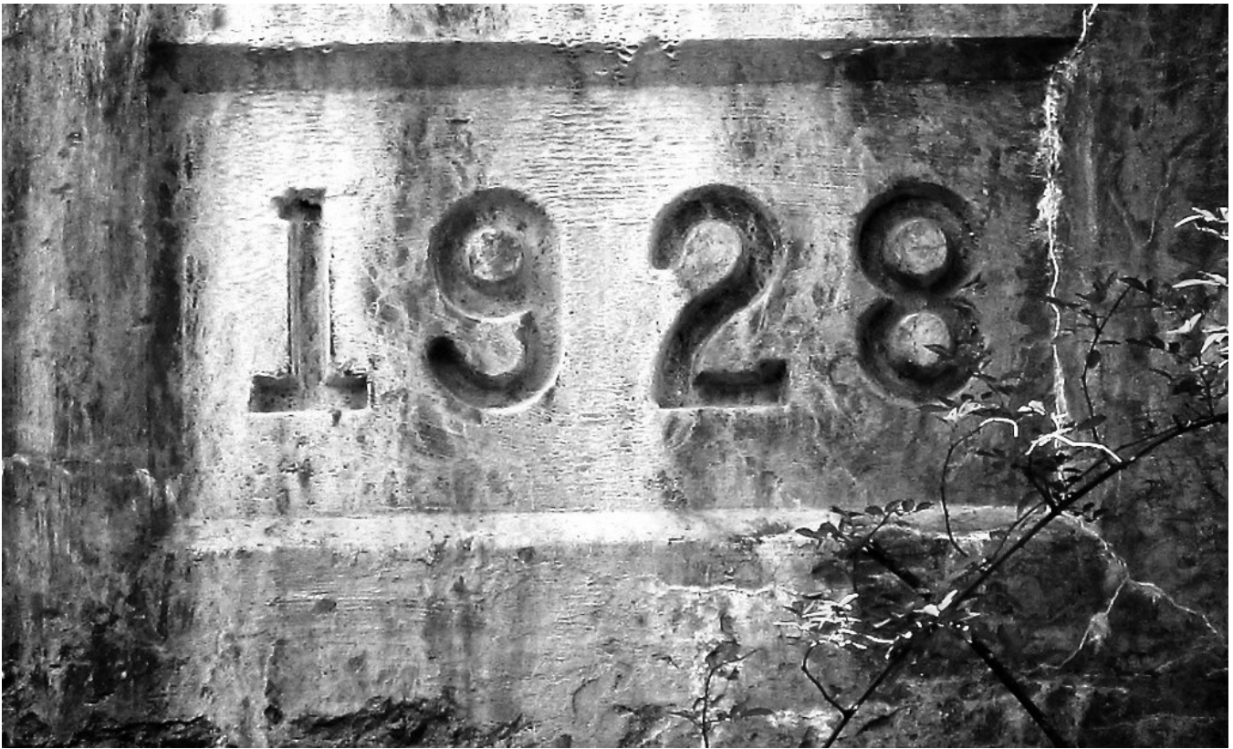
8. central steam plant masonry unit, fitchburg
