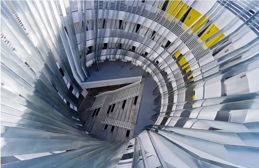
Figure 14: The building is inward-focused, with a central atrium and gathering space defining the character of the living area. Sheet metal fins add visual interest while hiding services and providing structural support.
