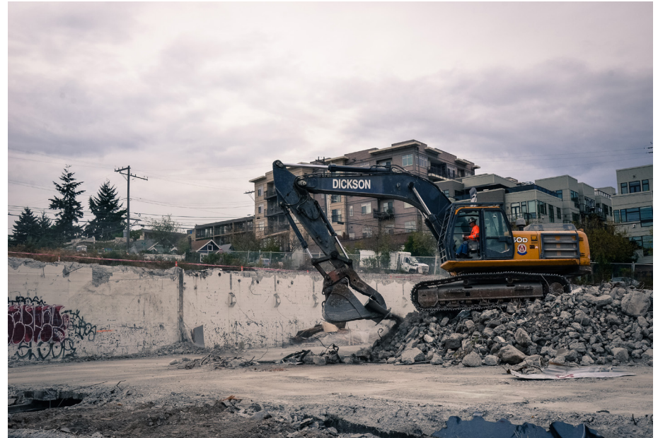
Figure 30: demolition of the existing building began summer 2014.
