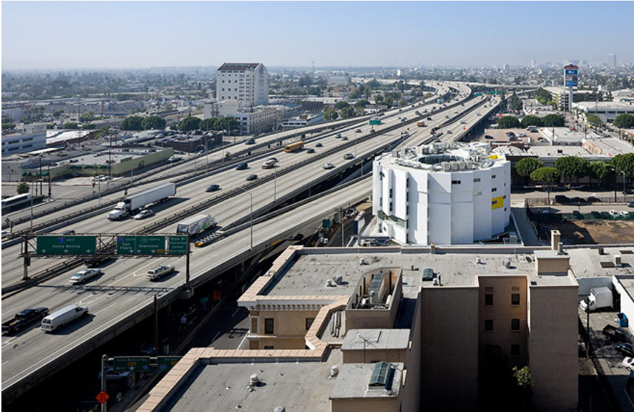
Figure 13: The New Carver Apartments are a response to the car-dominated site, an abstract form that helps deflect noise that would disrupt the quality of life within.
