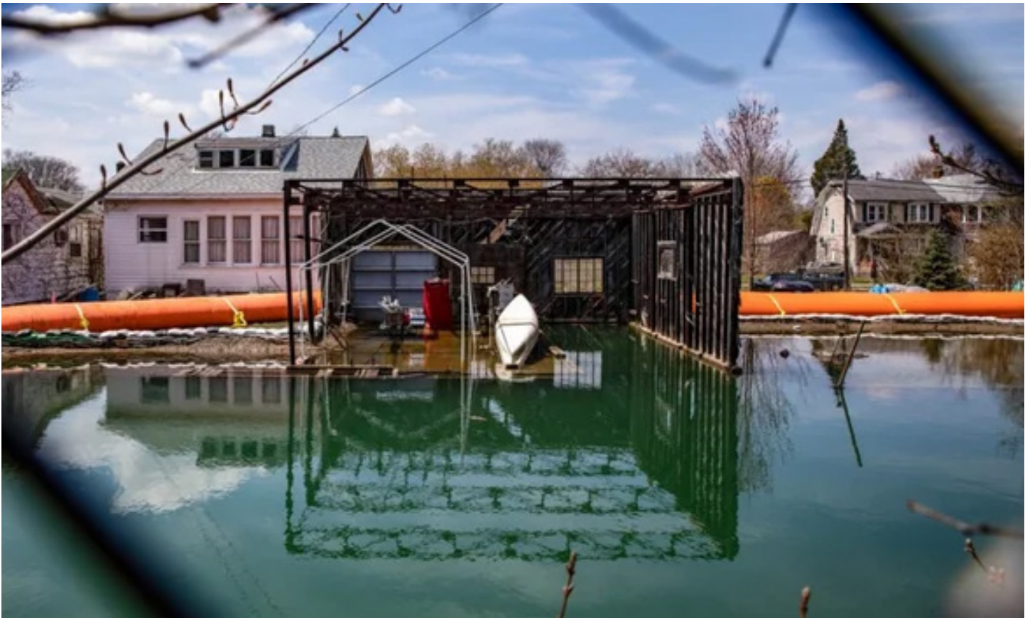
Inflatable Tiger Dam Flood Control Measures Planet Detroit, Photographer: Demetrio Nasoi
