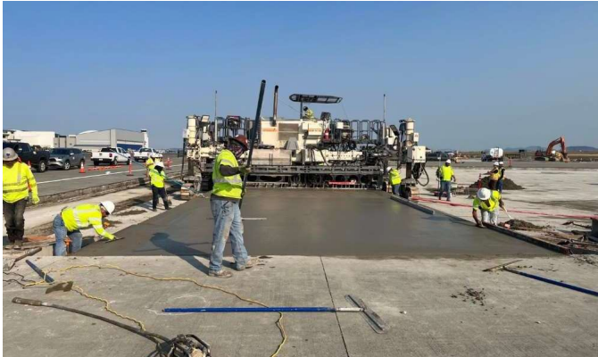
Figure 19 – NASWI Finishing Concrete
