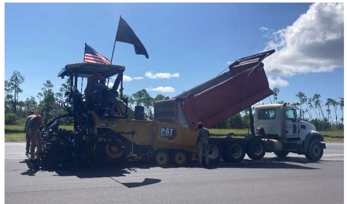
Figure 27 – TAFB Asphalt Transfer to Paver
