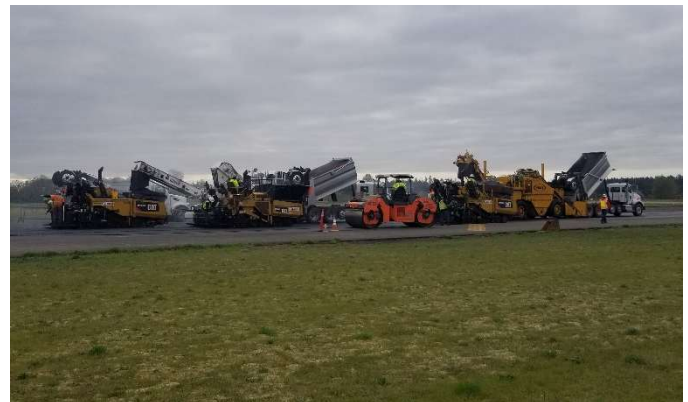
Figure 17 – JBLM Three Pavers in Tandem
