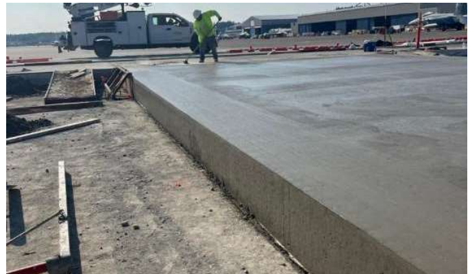
Figure 22 – NASWI Fresh Concrete
