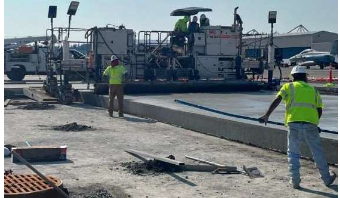
Figure 20 – NASWI Concrete Paving Operations
