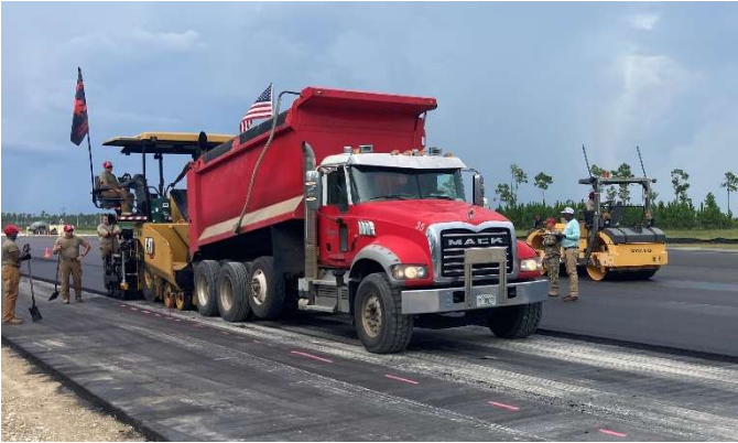
Figure 24 – TAFB Paver, Dump Truck, and Roller
