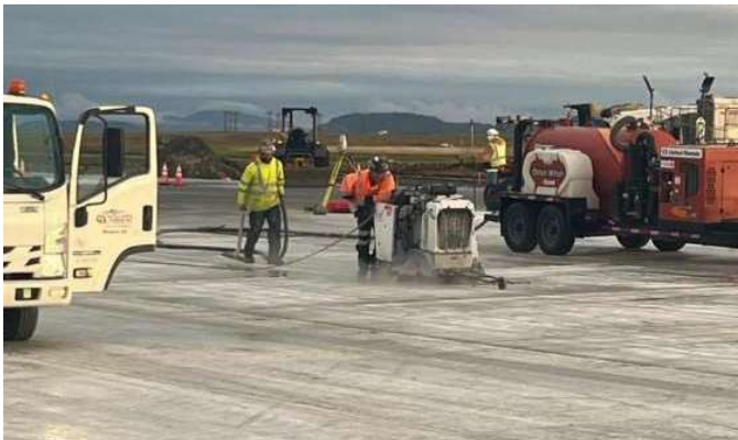
Figure 21 – NASWI Saw Cutting Expansion Joint
