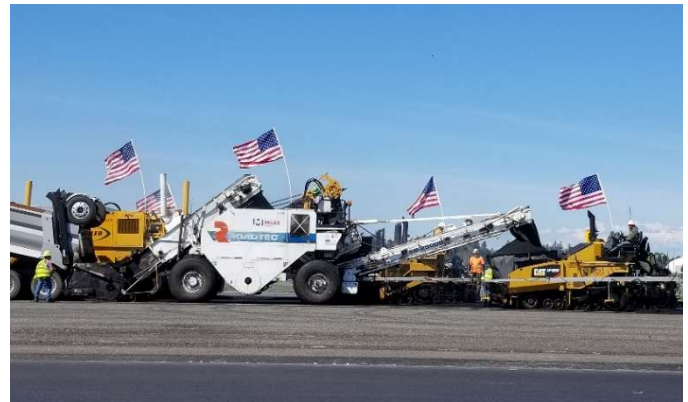
Figure 15 – JBLM Dump Truck, MTV, and Paver
