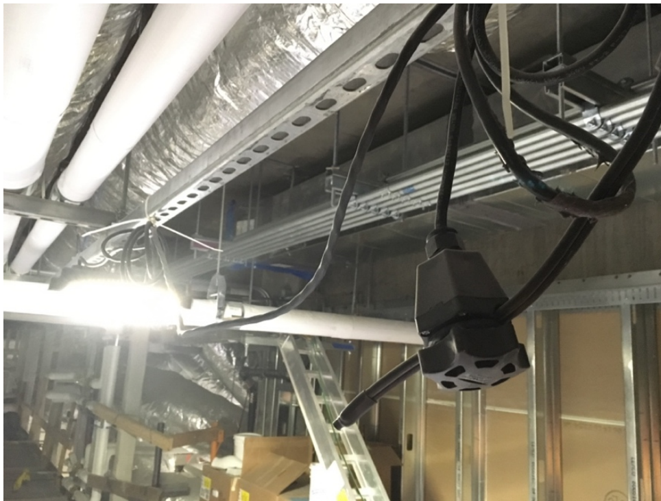
Figure 19: FM10 and Twist-Lock Connector in Interstitial Area
