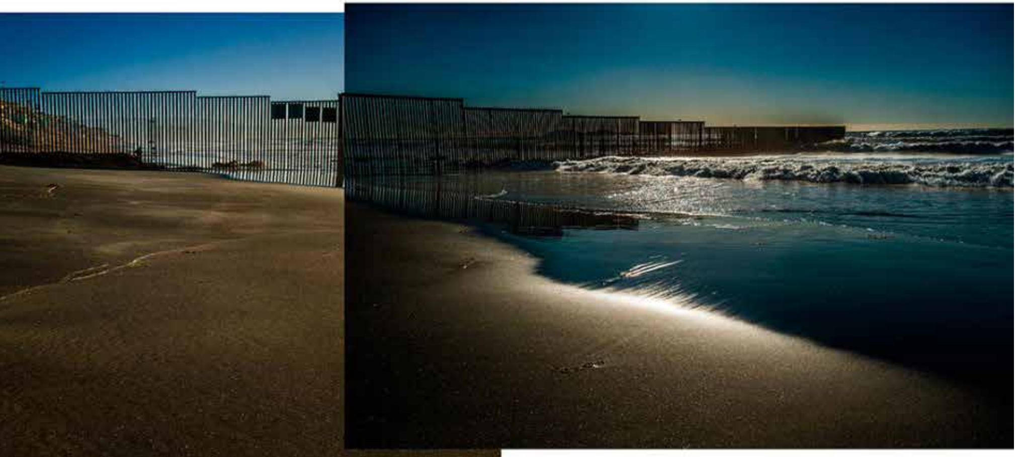
Figure 18: Border wall at the San Diego and Tijuana border meeting the ocean
