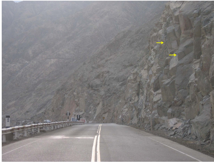
(a) Blocky slope with indications of missing rock blocks where toppling, sliding, and slumping failure modes are suspected.
