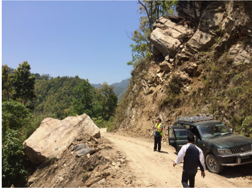
Figure 1.1: Rockfall during 2015 Gorkha earthquake in Nepal
