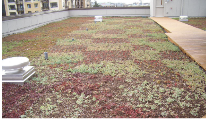
Figure 1. Extensive Green Roof Example. Seattle Cancer Care Alliance roof. Photo Credit: Annika McIntosh, 2009
