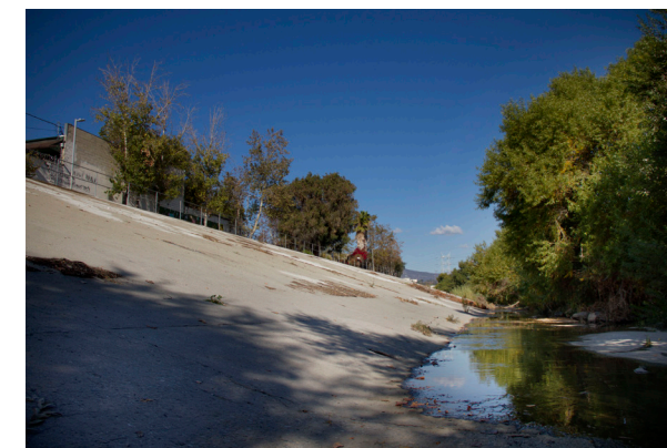
figure 30. Knox Avenue facing the storm concrete barrier at the river.
