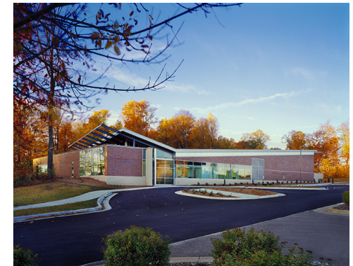
Figure 52: Johnson Creek Exterior Image Courtesy of Cannon Design
