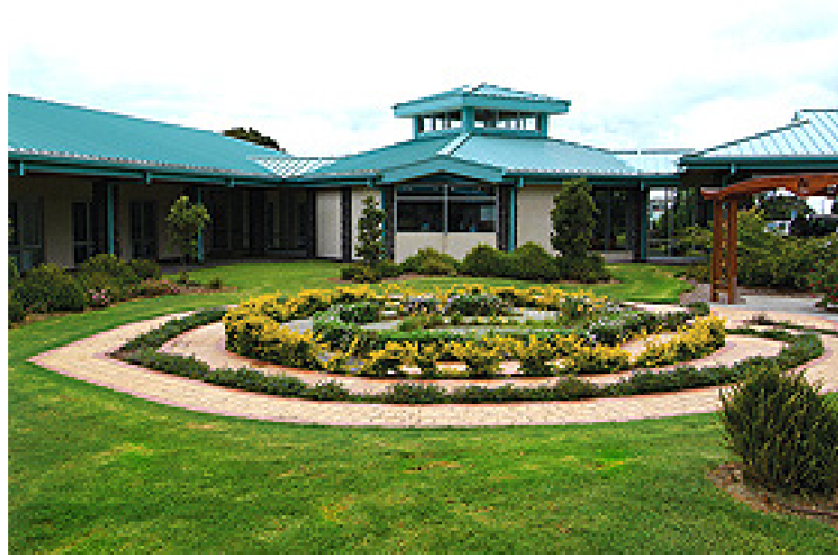
Figure 70: North Hawaii Hospital Exterior Healing Gardens
