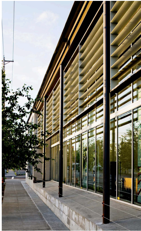
Figure 46: North Portland Clinic Entry Image Courtesy of Mahlum
