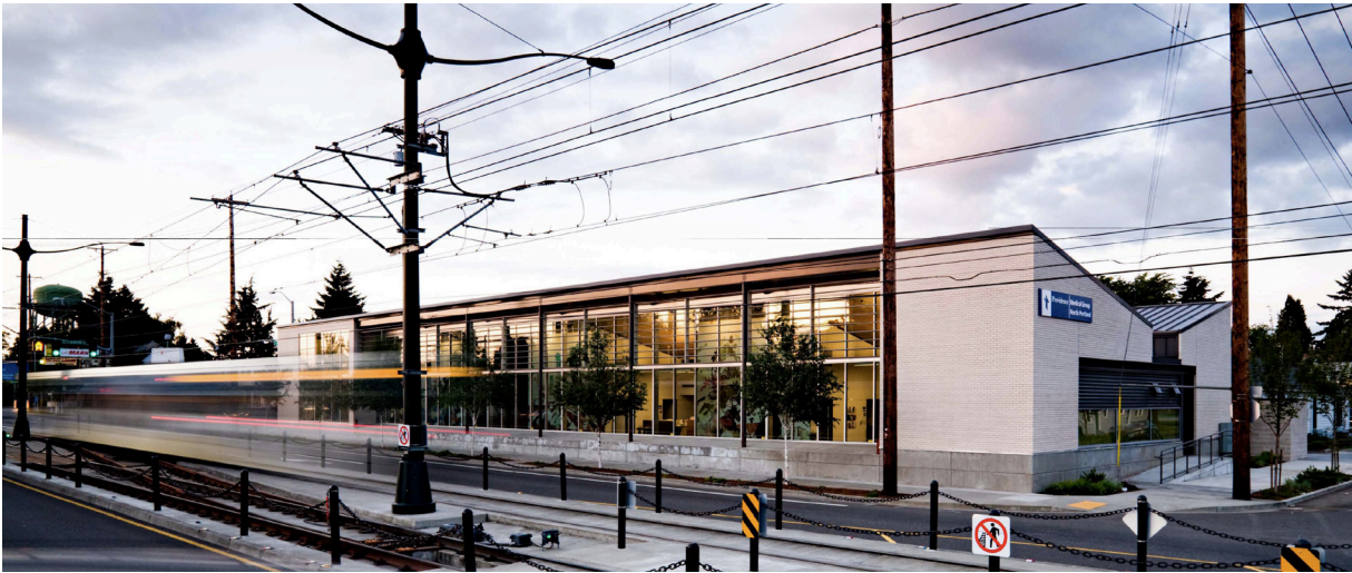
Figure 43: North Portland Clinic Exterior Image Courtesy of Mahlum
