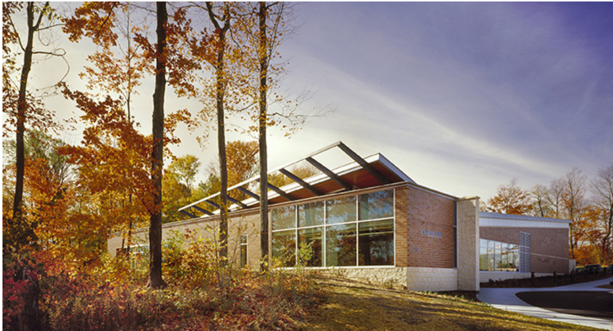
Figure 51: Johnson Creek Exterior Image Courtesy of Cannon Design
