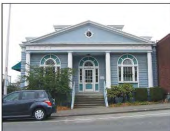
Columbia Lumber Company Office
