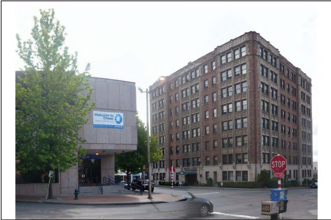
[FIG 3.11] Site Photos of South entrance of the Plaza
