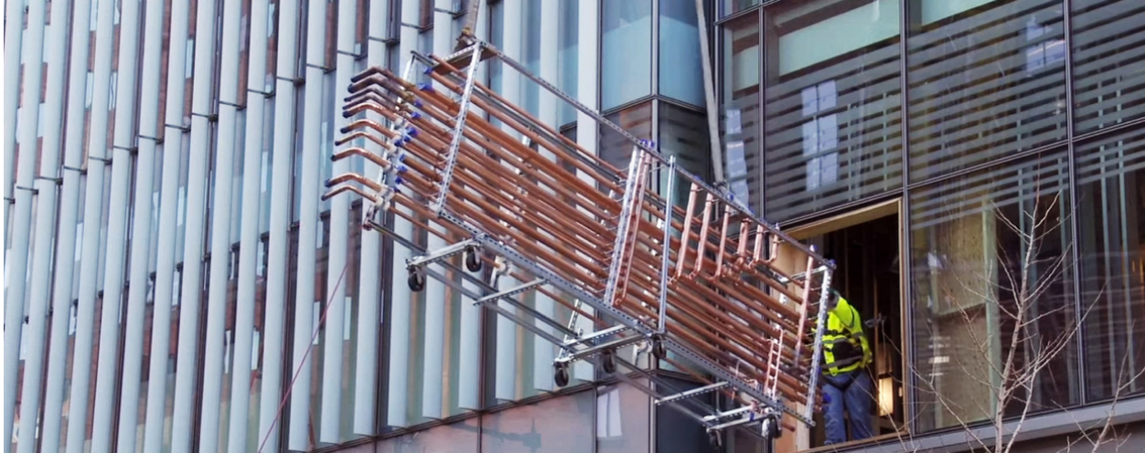
Figure 13. Delivery of a prefabricated utility rack. Source: (Teichloyz, Sarma et al. 2017).
