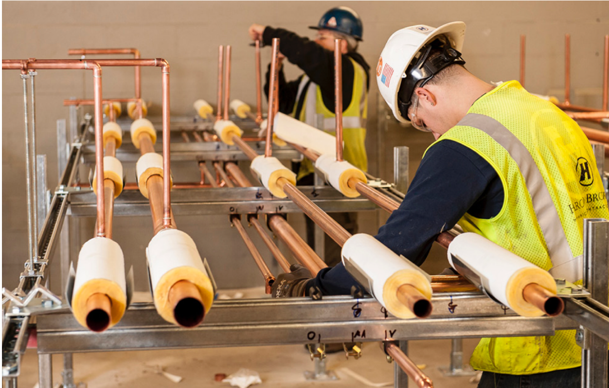
Figure 12. Prefabrication of plumbing racks at Consigli’s Prefab Lab. Source: (Teichloyz, Sarma et al. 2017).
