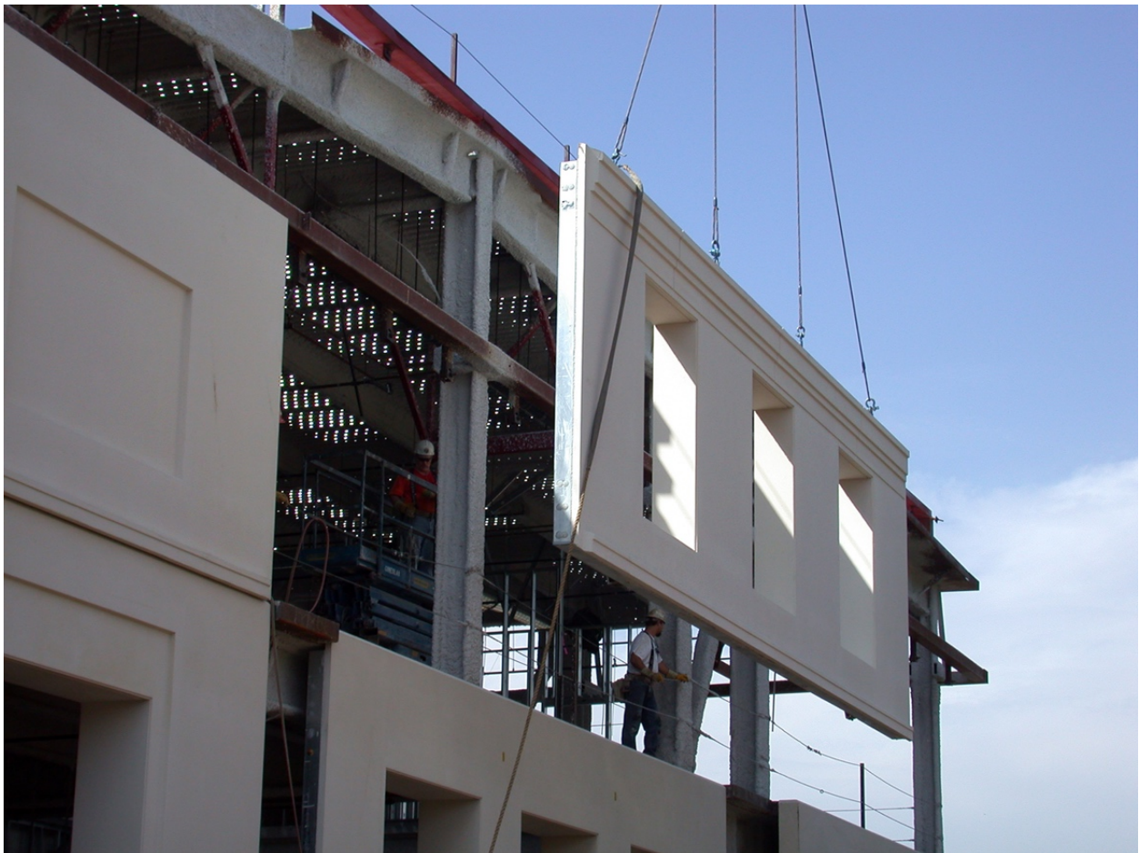
Figure 32. Precast wall panel being hoisted in place. Source: National Precast Concrete Association (NPCA). Retrieved from: http://precast.org/wp-content/uploads/2014/08/Precast-Concrete-Wall-Panel-Install.jpg .
