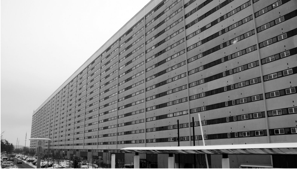
Figure 6. Le Haut du Lièvre, Nancy, France, by Bernard Zehrfuss (1960). Retrieved from: http://www.enattendantmieux.org .
