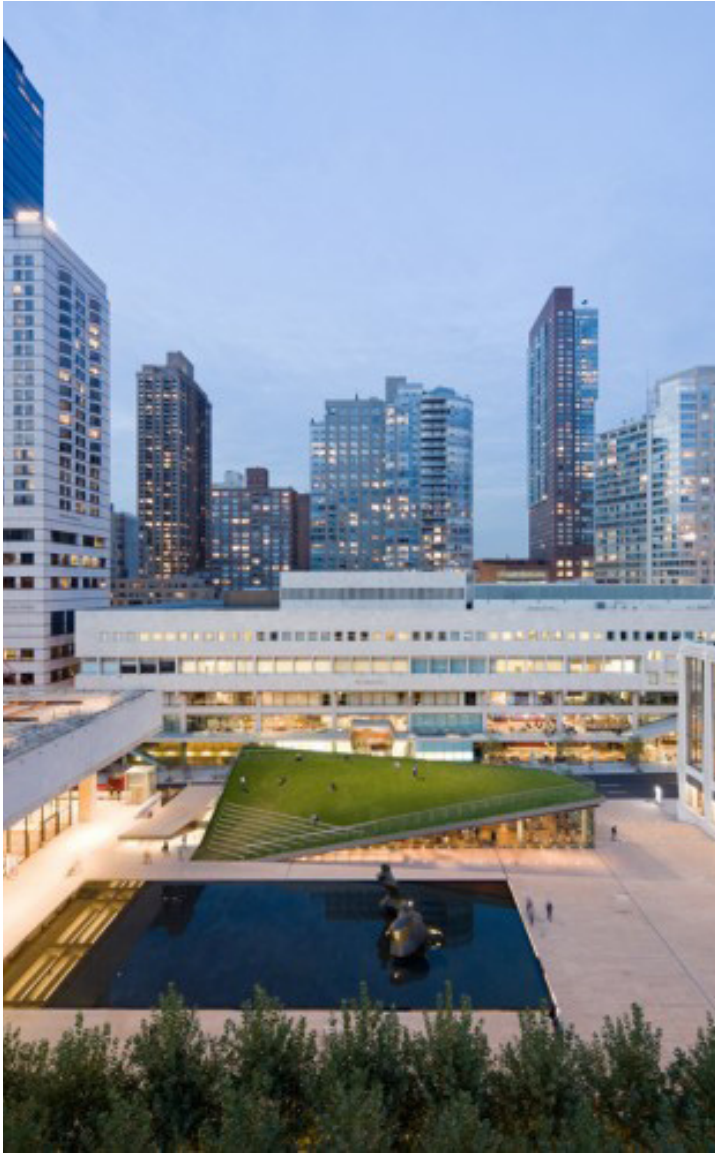
Figure 47: Lincoln Center Hypar Pavilion, DS+R
