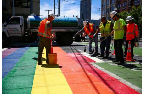
Figure 2.1. SDOT crew painting a Community Crosswalk, Capitol Hill, Seattle. photo: Joshua Trujillo/Seattlepi.com ("Seattle Celebrates" 2017)
