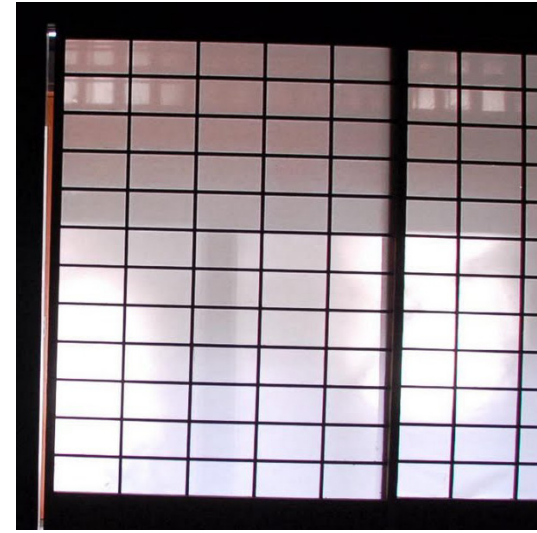
b : 3'x 8' - .2 mm laminated shoji paper in 2"x 2" red cedar frames
