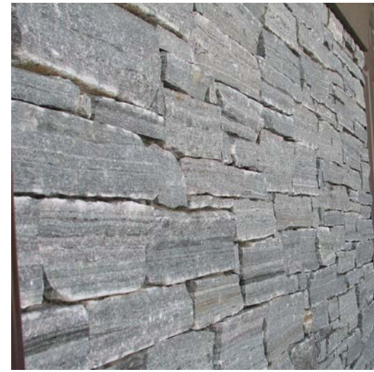
b : 6''x 3''x 36'' granite block ledgestone walls
