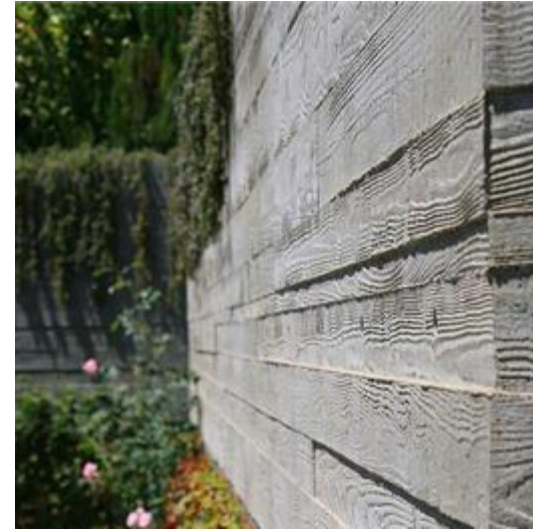
c : board-formed concrete terraces
