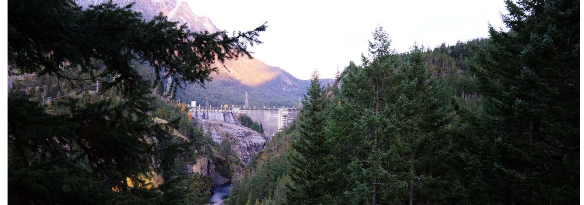
Figure 1. Photograph of Diablo Dam from the west.
