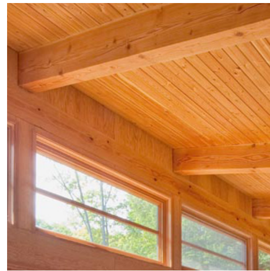
a : 2"x 6" clear stained red cedar decking and 6"x 6" rough sawn red cedar beams
