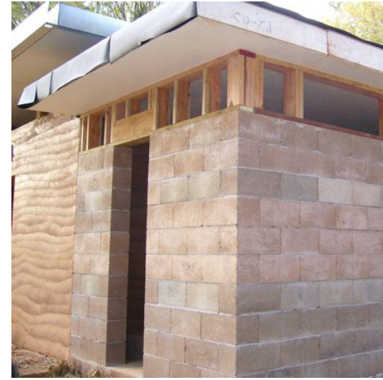
b : 6" rammed earth wall and 8"x 8"x 16" soil composite cmu blocks
