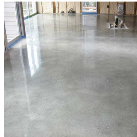
c : 12" site-cast polished concrete slab
