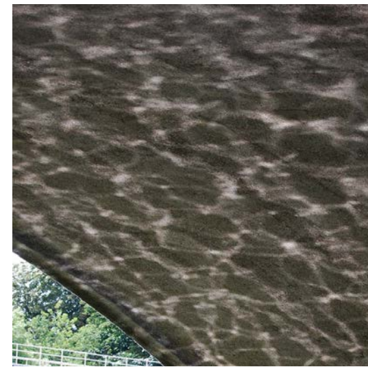
a : 6'' pre-cast concrete slab roof
