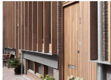
C. Intensive use of wood on the ground floor
