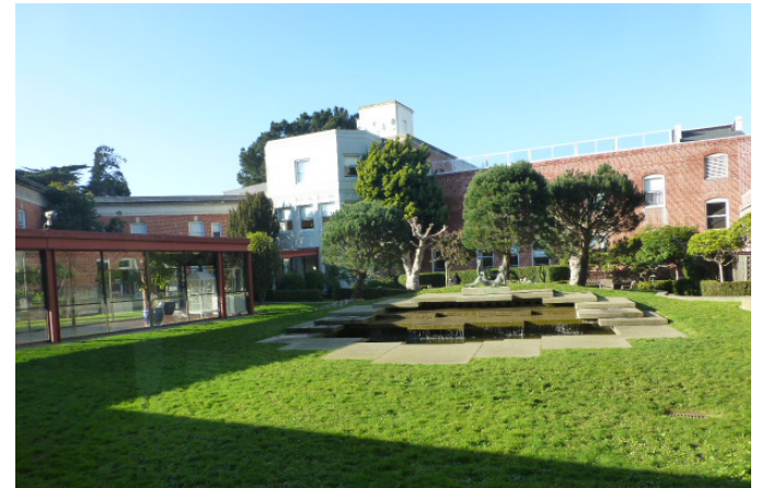
JHSF GOODMAN BUILDING GROUND FLOOR COURTYARD AND FOUNTAIN
