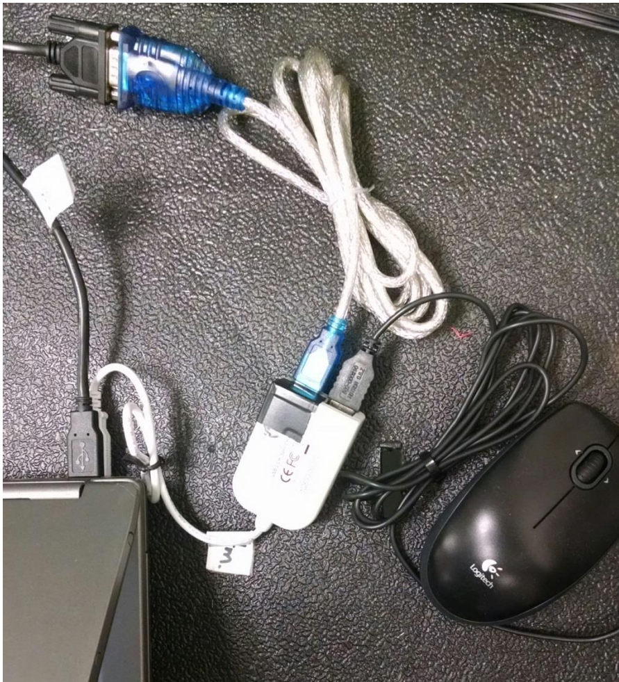
Figure III.4. – Laptop data and electrical connections.
