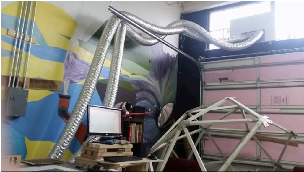
Figure 5. Added ducting for the laser cutter. Photo by Tony Loiseleur.
