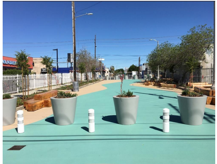
Figure 3.5 Image of cool pavement in a Los Angeles community.
