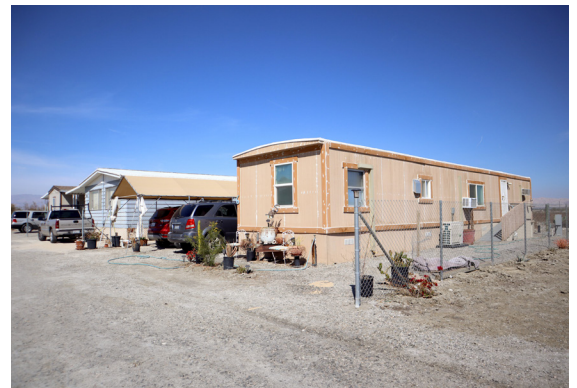
Figure 5.12 Image mobile homes on site.
