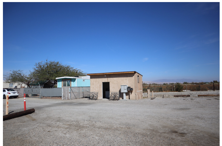
Figure 5.22 Image of existing laundry room and surrounding conditions.
