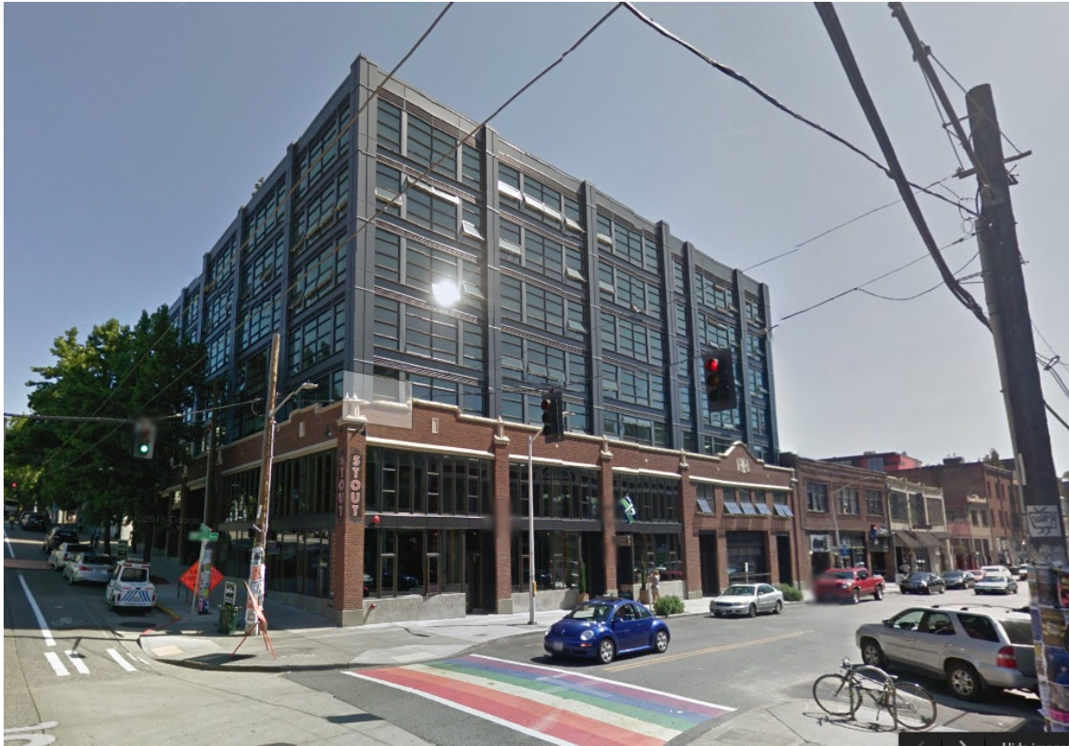
Figure 5. Sunset Electric Apartments, 1530 11th Ave (Image Google Earth, August 2015)
