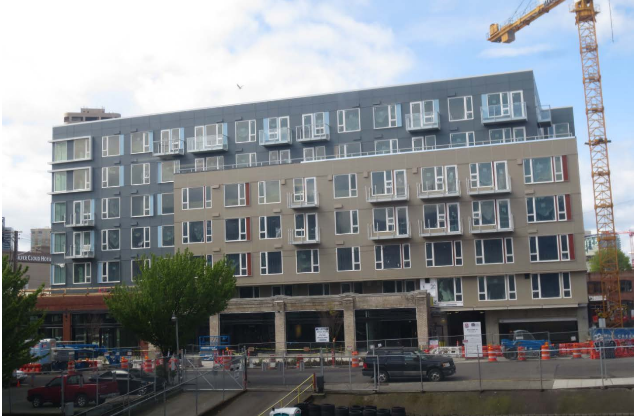
Figure 6. 1414 10 th St, very little historic fabric left to these two character structures (Image: Manish Chalana)
