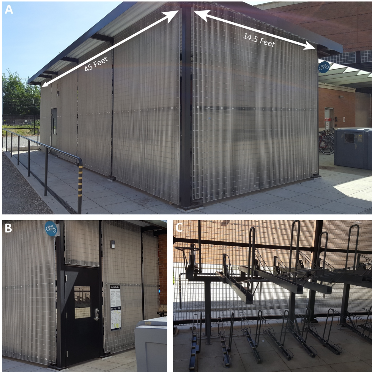
(A) This bicycle cage was added to Sound Transit's Beacon Hill Link station in 2016. It has capacity to securely store 48 bikes in a footprint of 14.5 x 45 feet, requiring less than half as much space per bike as bicycle lockers. (B) Entry is controlled by keycode access and provides a record of every person who accesses the bike cage. (C) Double-decked racks help make the best use of space inside the bike cage. Photos by author, April 30, 2016.
