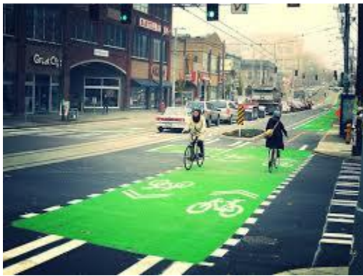
Figure 13. Example of Class 2 bicycle facility, a two-way protected bicycle lane. Source: seattle.gov
