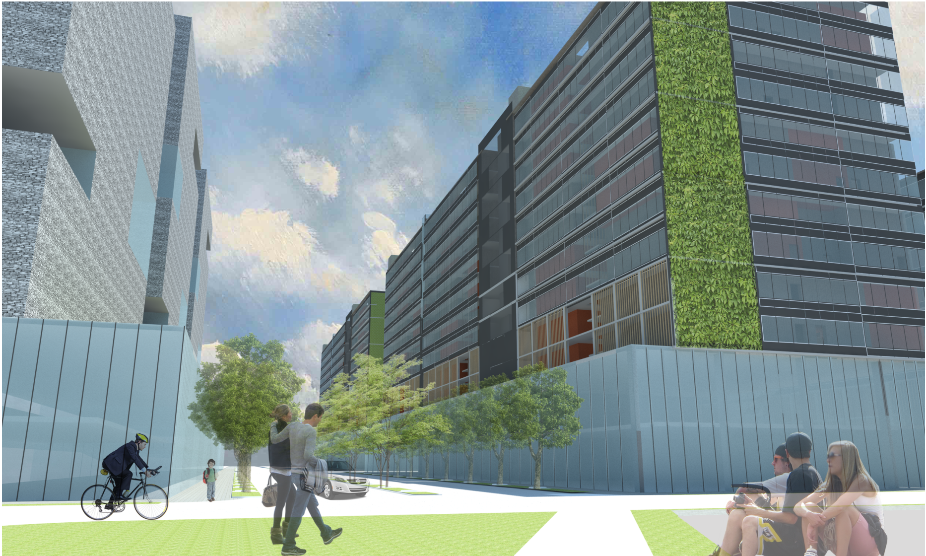
Figure 30. Retail street view.
