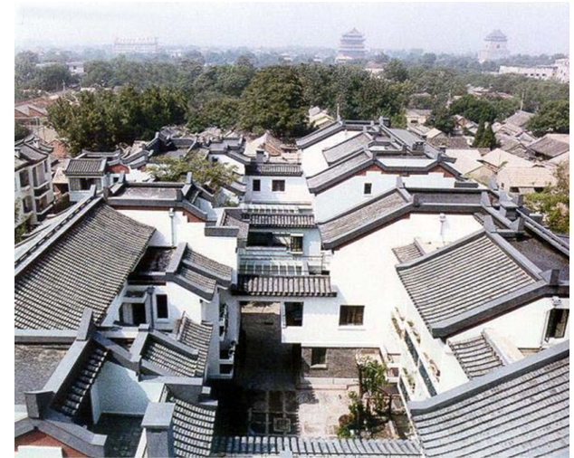
Figure 16. Juer Hutong Project 1.
