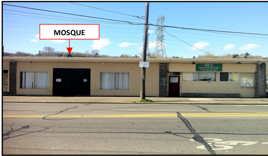
Figure 29: Façade of mosque and adjacent Oromo Cultural Center office
