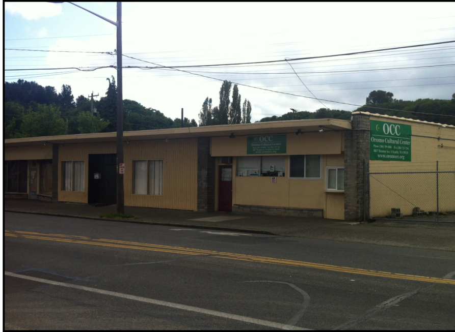
Figure 32: Oromo Cultural Center, looking southwest. The façade has not changed substantially over the years in comparison to the historic photograph in Figure 27, though some of the large commercial windows are partially covered now. Note the exterior sign placement on the sidewall, on the right of this photo is the same, 63 years later.
