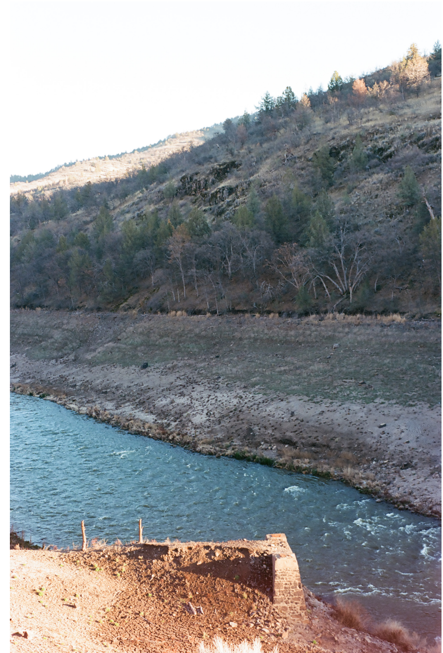
Fig. 1 Foundation at the Narrows, 2025
