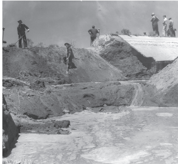
Fig. 4 Men building diversion canals from the Klamath River in 1933. Source: Oregon Historical Society
