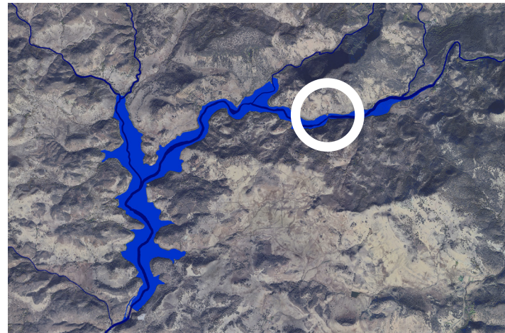
Fig. 6 Klamath River with Iron Gate Reservoir filled, site indicated, and river path indicated.
