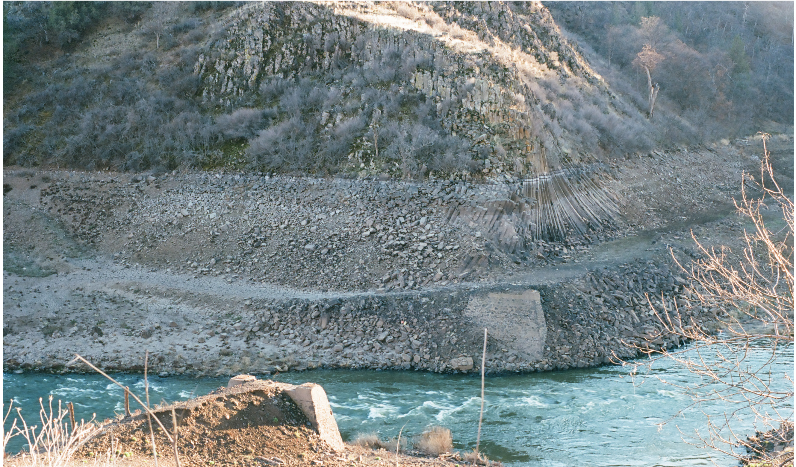
Fig. 9 Site for bridge design with both foundations in view. Basalt columns on the opposite side of the river are stained by the height of the reservoir that is now drained.
