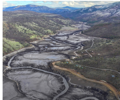
Fig. 17 Iron Gate Reservoir immediately after dam removal. Source: Swiftwater Films.
