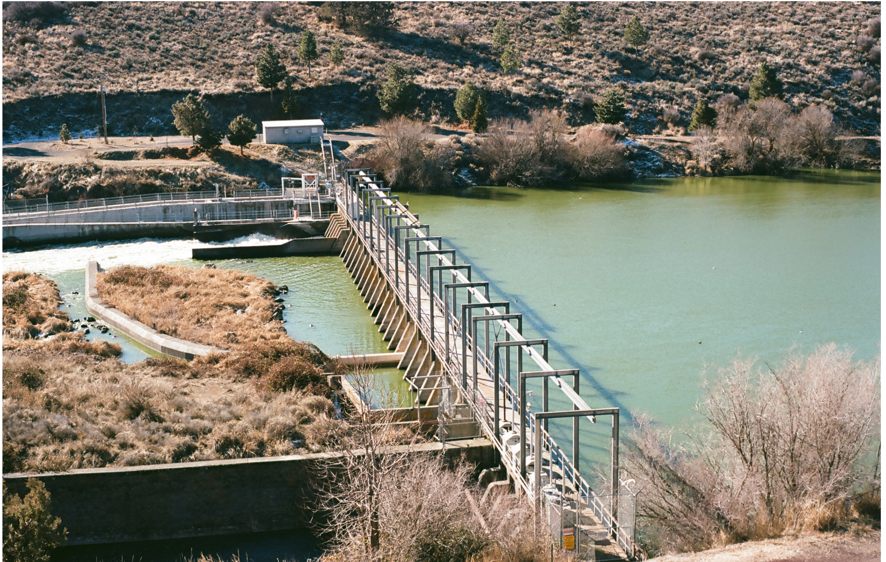
Fig. 19 Link River Dam, near Klamath Falls, OR. The last remaining dam on the Klamath River.
