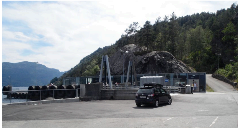
FIGURE 17. ROPEID TERMINAL IN CONTEXT NEXT TO GRANITE CLIFF FACE.
