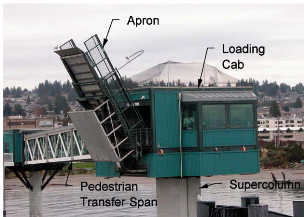
FIGURE 14. SUPERCOLUMN PEDESTRIAN TRANSFER SPAN, EDMONDS.
