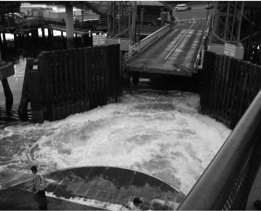
FIGURE 4. FERRY APPROACHING WING WALLS AND VEHICLE LINKSPAN.
