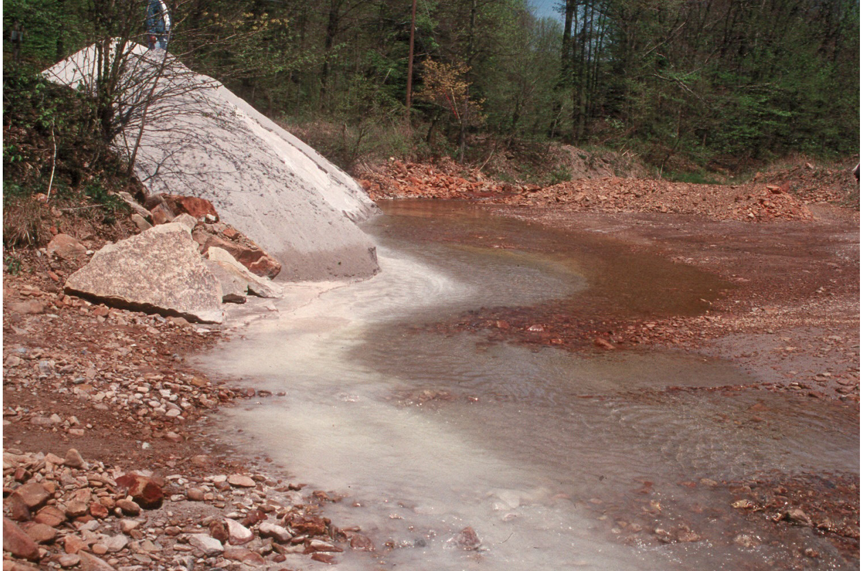
Figure 4: Image of Acidic Water Treatment
