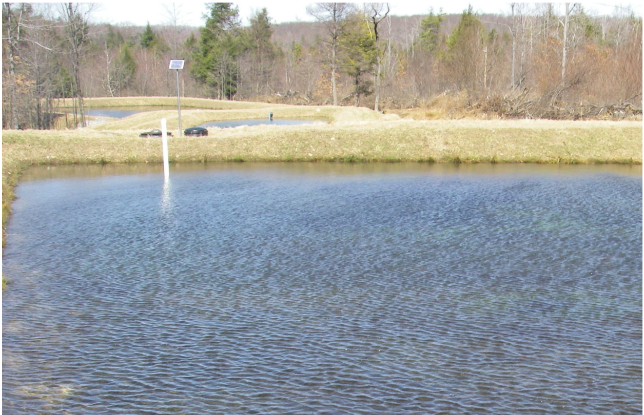
Figure 5: Image of Acidic Water Treatment
