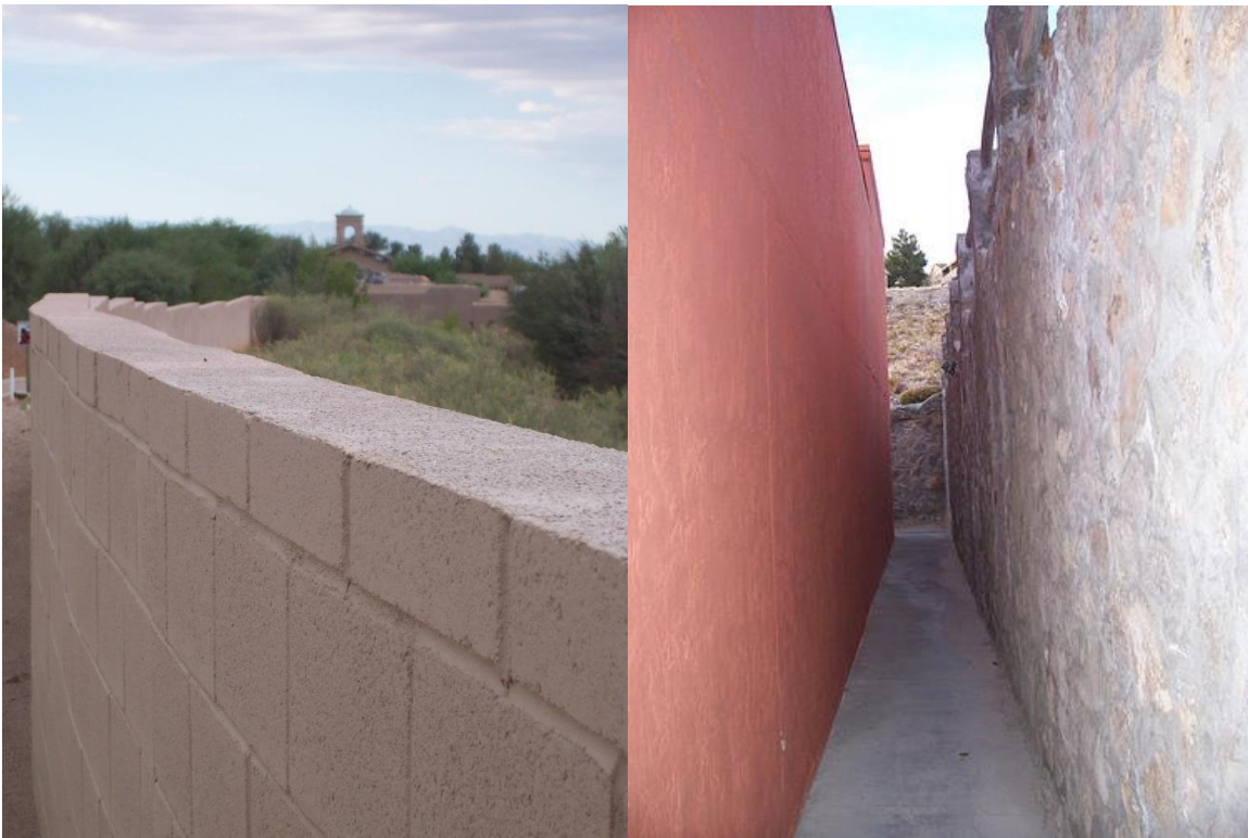
Figures 20 and 21. Walls near gated communities, adjacent to the border.
