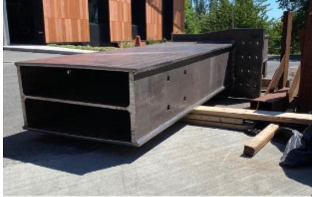
Figure 3.7 Sliding beam
