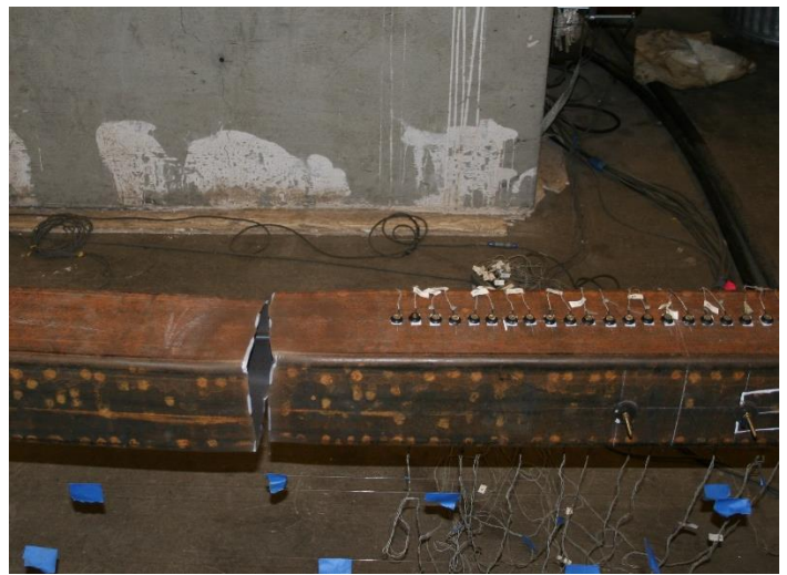
Brace Fracture: 1.16" T1 cycle
