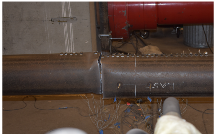
Brace Fracture: 1.75" T2 cycle
