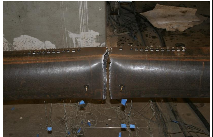
Brace Fracture: 2.54" T1 cycle
