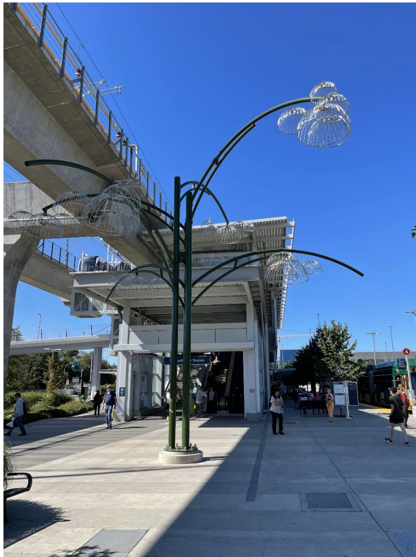
Figure 8: Northgate Transit Center
