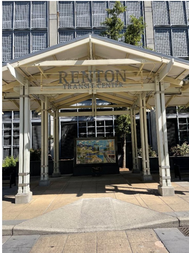
Figure 7: Renton Transit Center
